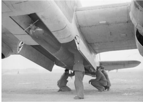
Figure 11 RAF Coastal Command, 1939-1945. Armourers loading a MK XII ariel torpedo into a Bristol Beaufort Mk 1 of No 42 Squadron. No 42 Squadron were stationed at RAF St Eval in 1941.
