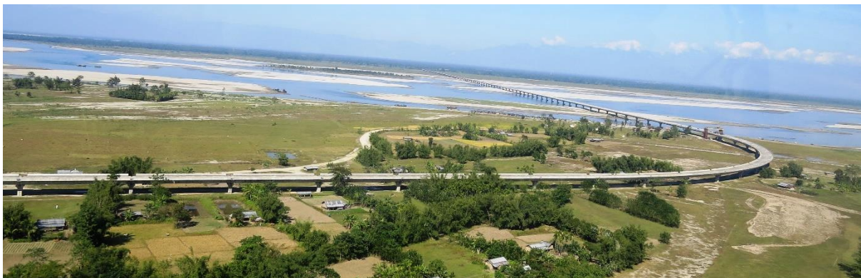
India's longest River Bridge
