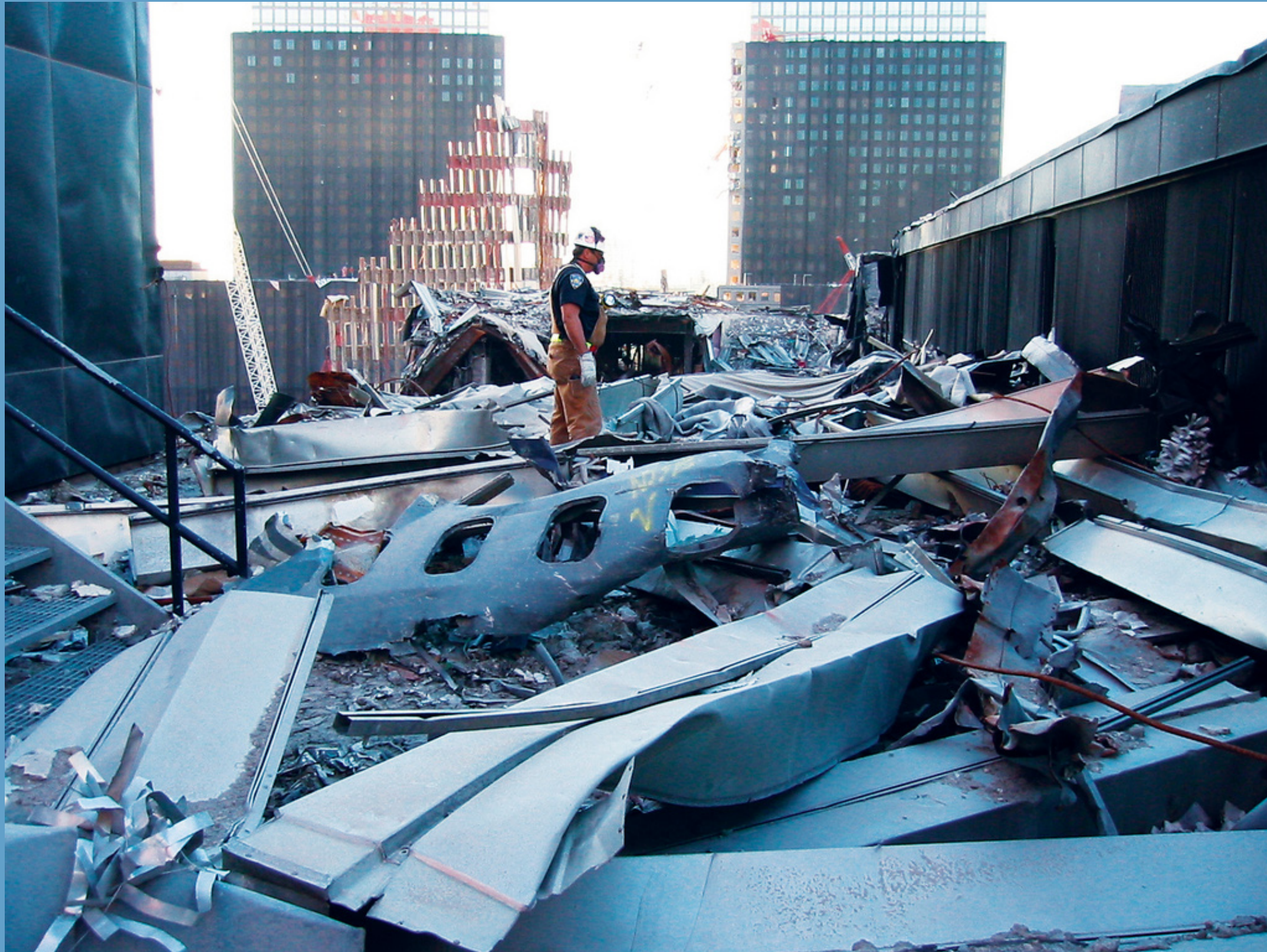
Aircraft fuselage found on the roof of Building 5
