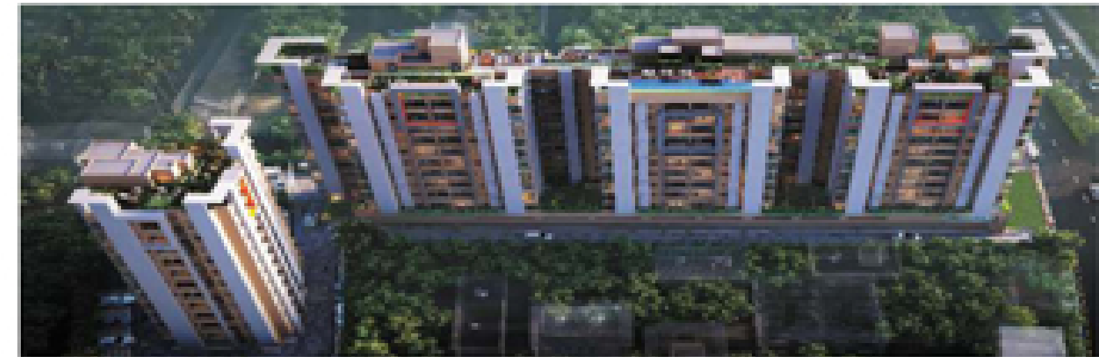
RISHI VENTOSO, Madhyamgram, Kolkata (Under Construction)
