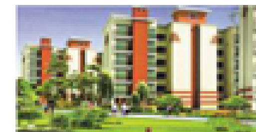
RISHI APARTMENTS*, Badli, Himachal Pradesh
