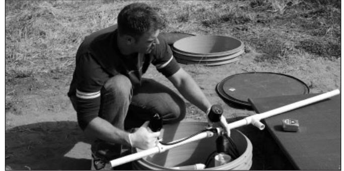
Raise the bottom float to stop the alarm. A yellow LED should light up.
