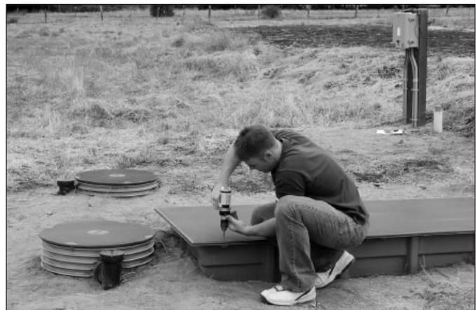
**WARNING:** If lid bolts are missing, replace them with spares. If you have no spare lid bolts, fasten the lid with a self-tapping screw, and immediately call your Dealer for replacement bolts. If the lid is unbolted or if the lid or riser are damaged, be sure to securely block access to the tank opening before leaving the site. Open tanks are hazardous, and children or adults who try to enter them may be seriously injured, asphyxiated, or drowned.
