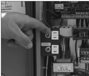
Release the switch back to the AUTO position. Make sure the pump comes on as the timer cycles. Timer cycles are shortened to about 30 seconds in test mode.
