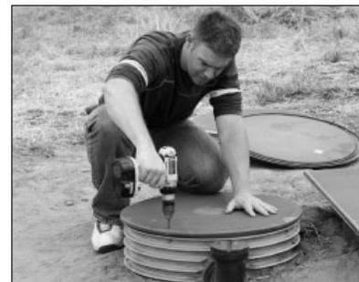
**WARNING:** If lid bolts are missing, replace them with spares. If you have no spare lid bolts, fasten the lid with a self-tapping screw, and immediately call your Dealer for replacement bolts. If the lid is unbolted or if the lid or riser are damaged, be sure to securely block access to the tank opening before leaving the site. Open tanks are hazardous, and children or adults who try to enter them may be seriously injured, asphyxiated or drowned.
