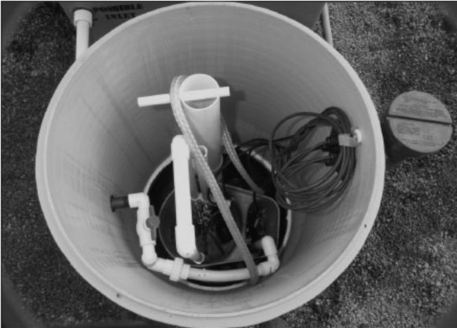
**Float assembly mounted in Biotube® vault.**
