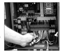
**WARNING:** Failure to identify a loose wire may cause intermittent failures, inconsistent panel operation and overcurrent conditions on the pumps.
