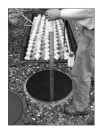
**NOTE:** Turn the laterals in the AdvanTex® treatment unit 180 degrees (so the spray nozzle turbines face up) prior to flushing to prevent nozzle clogging while material is being pushed along the lateral to the flushing valve.
