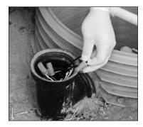
**WARNING:** Failure to use waterproof wire nuts can cause intermittent or permanent float failure.
