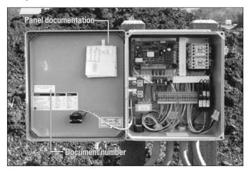
The system may have multiple control panels. Identify if there are control panels on the section of the system that you are about to start-up.
