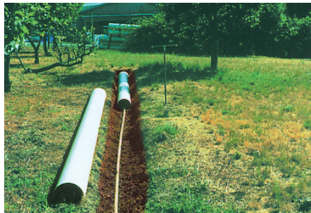
Shallow gravelless drainfield
