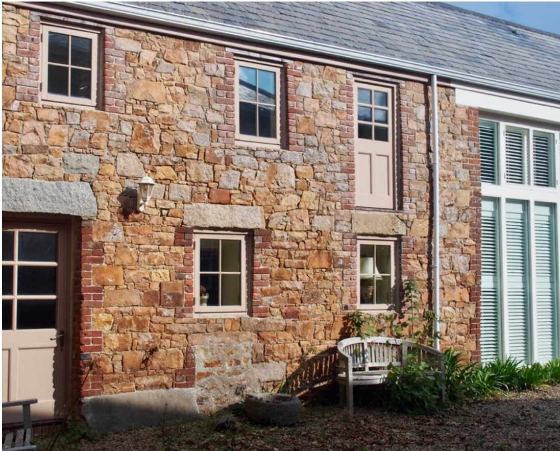
Oakdale courtyard buildings with original stonework now converted into apartments (2017)
