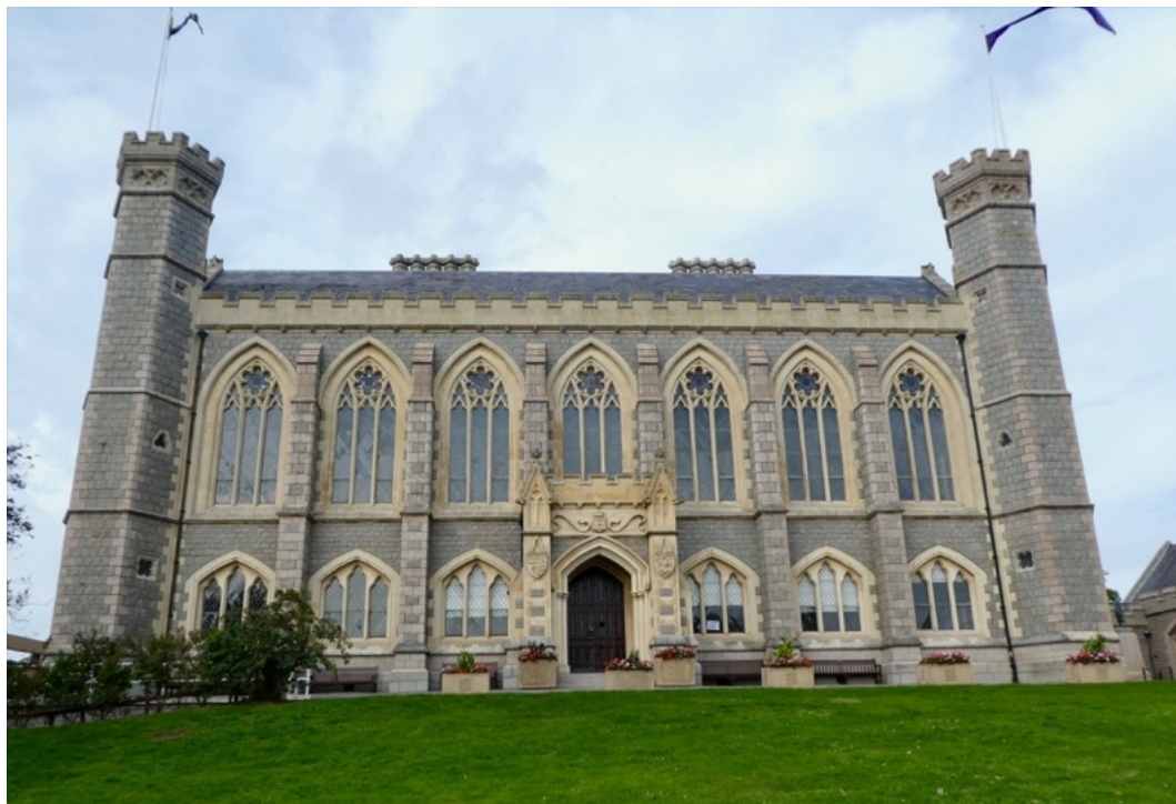
The main façade of Victoria College, Jersey (2017)
