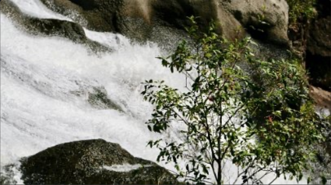
Spillway at Lake Baroon
