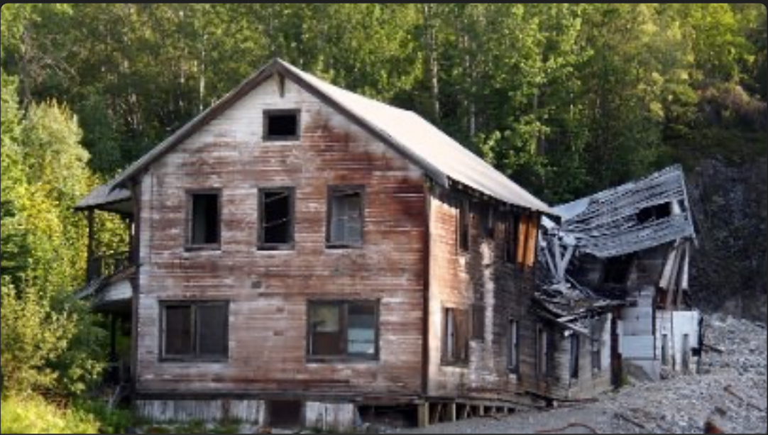
Kennicott Mine Buildings
