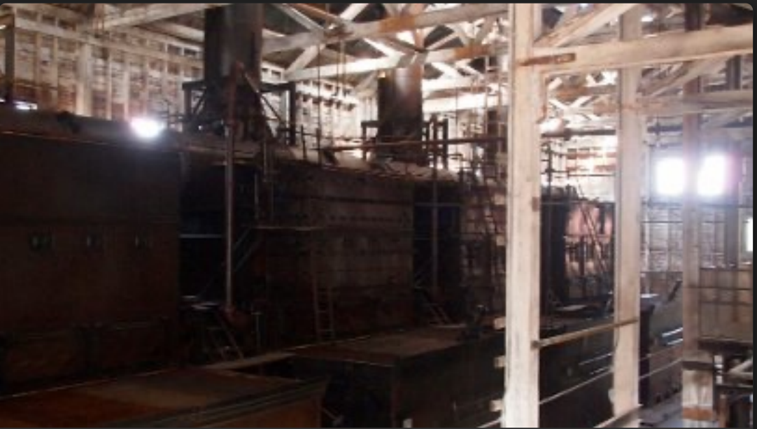
Kennicott Mine Buildings - Power Plant
