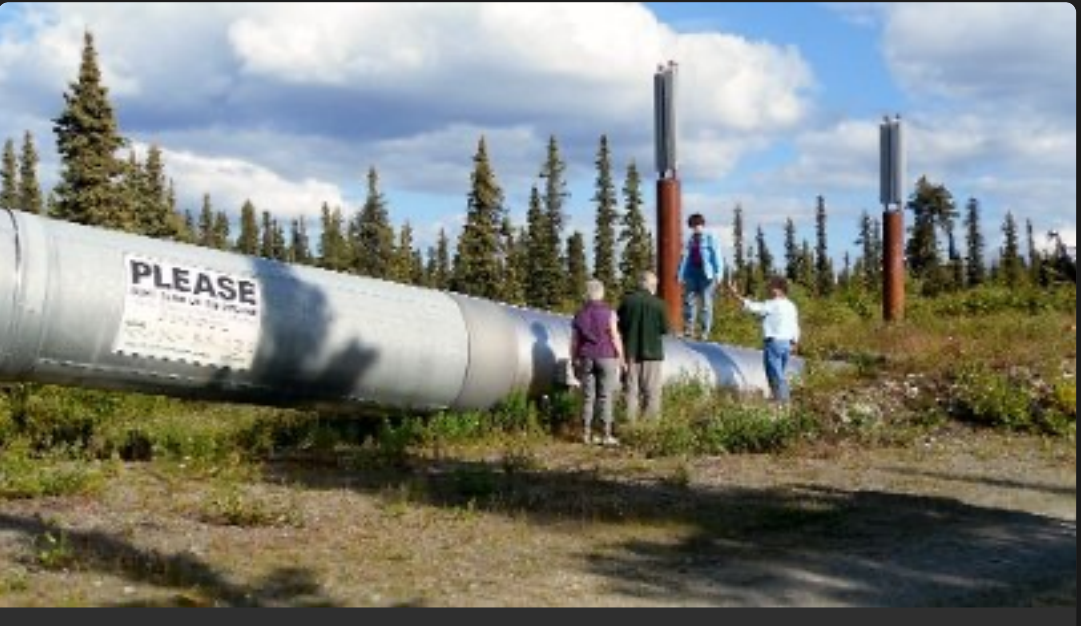
Trans Alaska Pipeline
