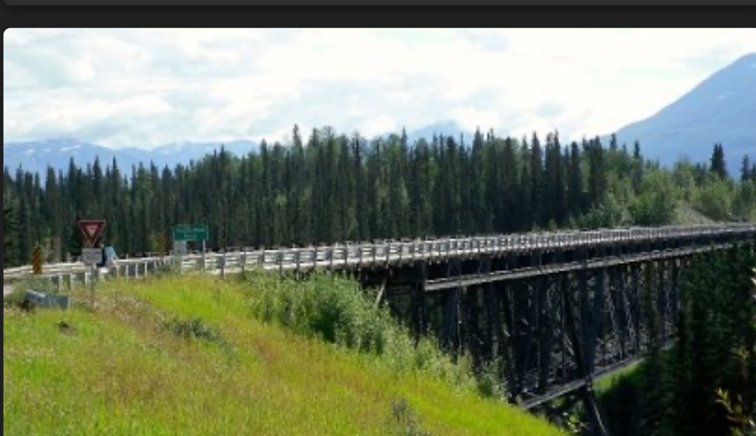
Road to McCarthy - Kuskulana River Bridge
