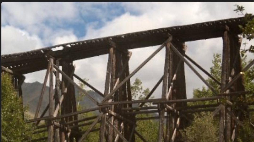
Road to McCarthy - old railway bridge
