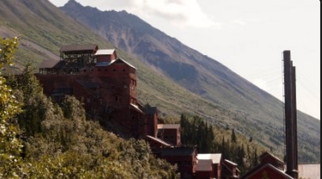
Kennicott Mine Buildings
