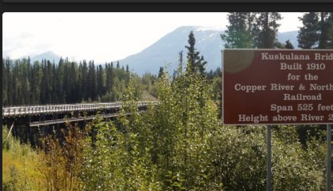
Road to McCarthy - Kuskulana River Bridge
