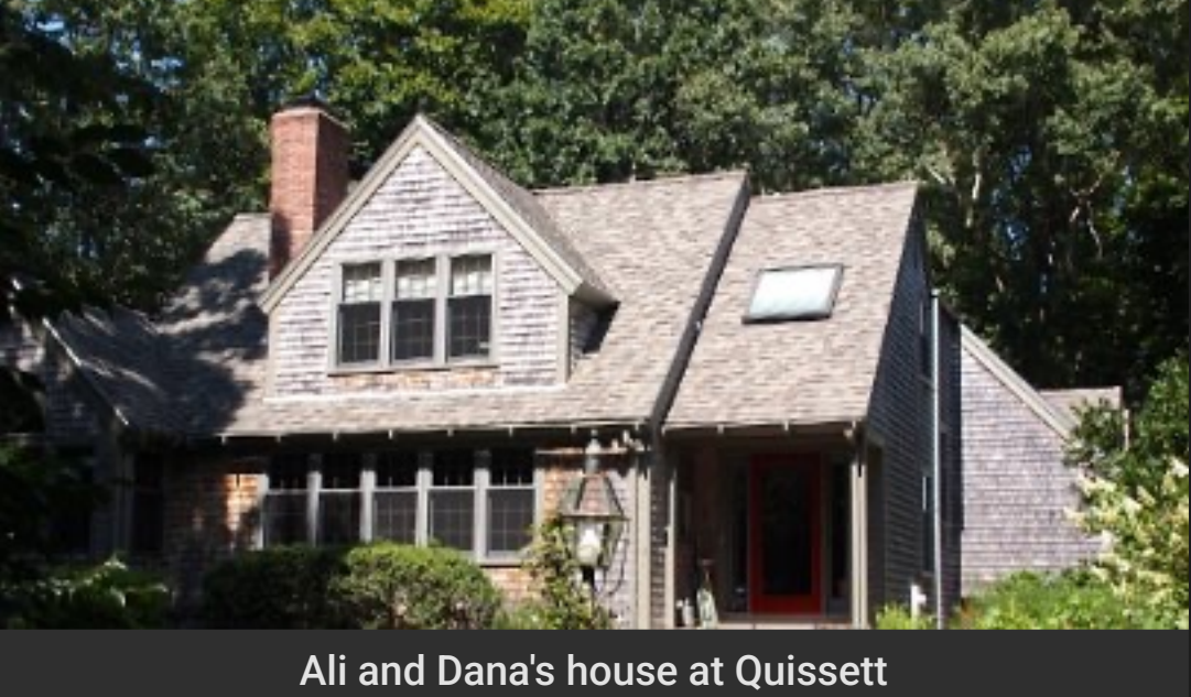
Ali and Dana's house at Quissett
