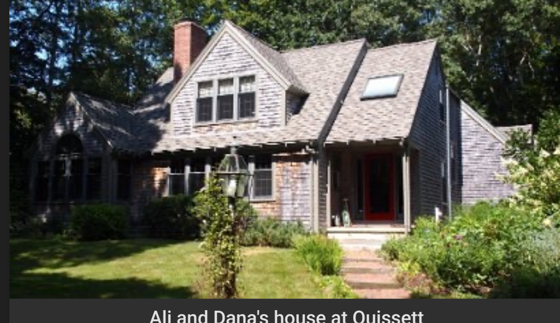
Ali and Dana's house at Quissett
