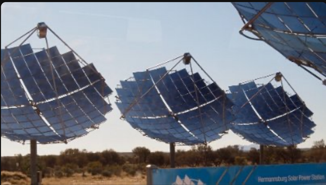
Hermannsburg solar power collection mirrors
