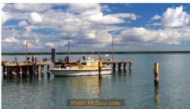
Weipa Harbour jetty
