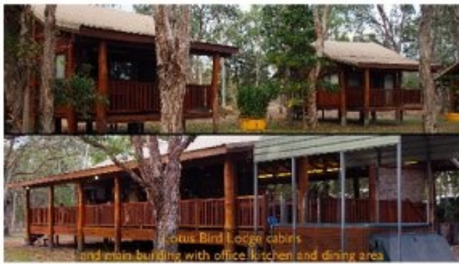
Lotus Bird Lodge Jabiru and main building with office kitchen and dining area
