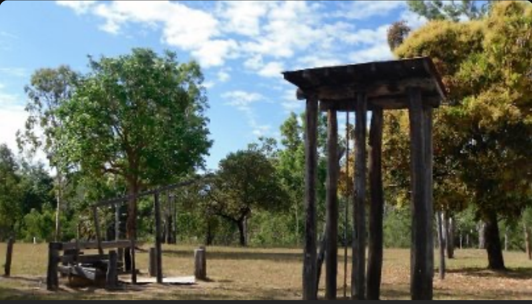
Old Laura Station water tank stand
