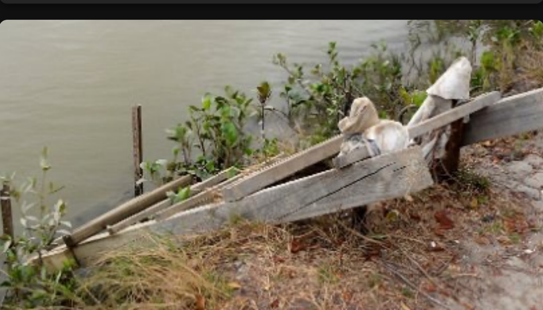
Annie River safety ladder
