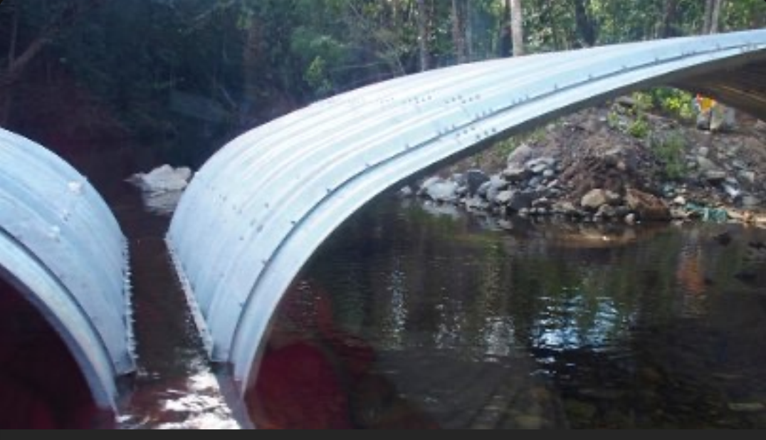
Bloomfield Track new bridge
