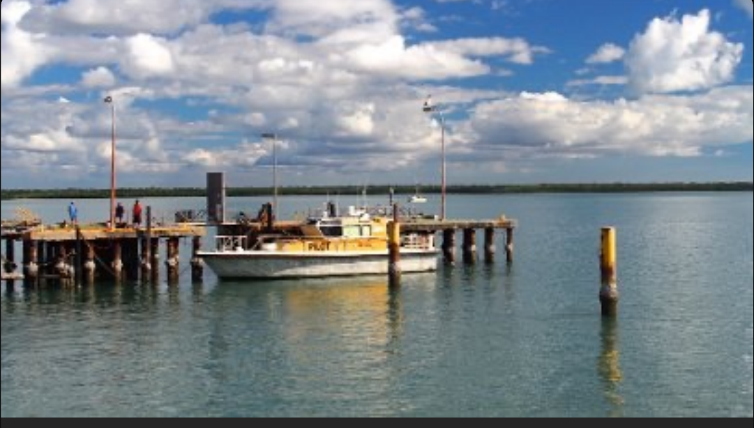
Weipa Harbour jetty
