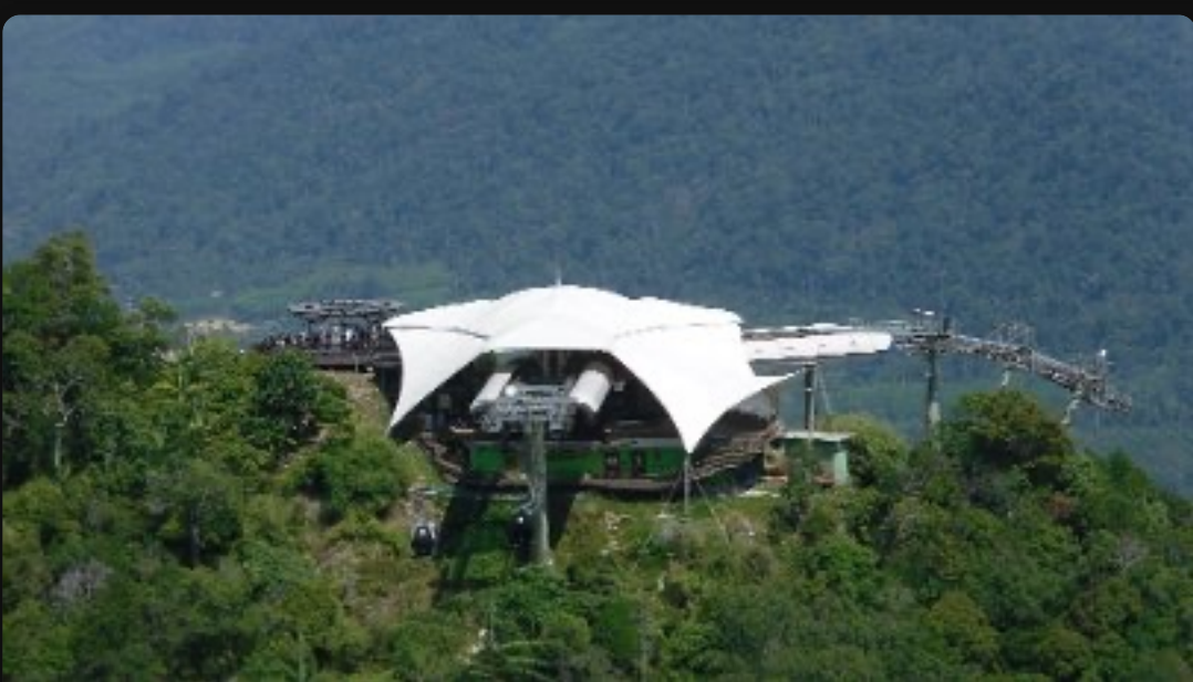
Cable car middle station from top station with gondolas
