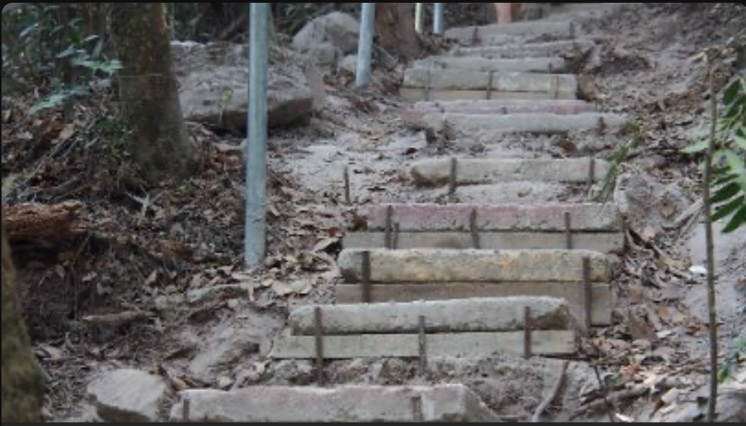
Temporary path to Skybridge on Gunung Matchinchang
