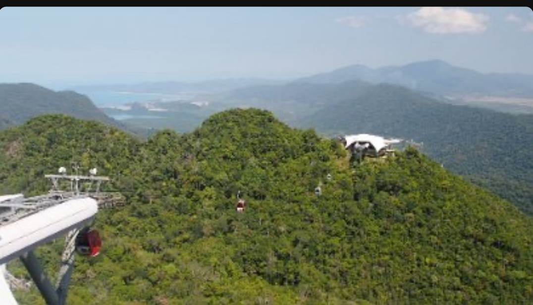
Cable car middle and top stations with view to north
