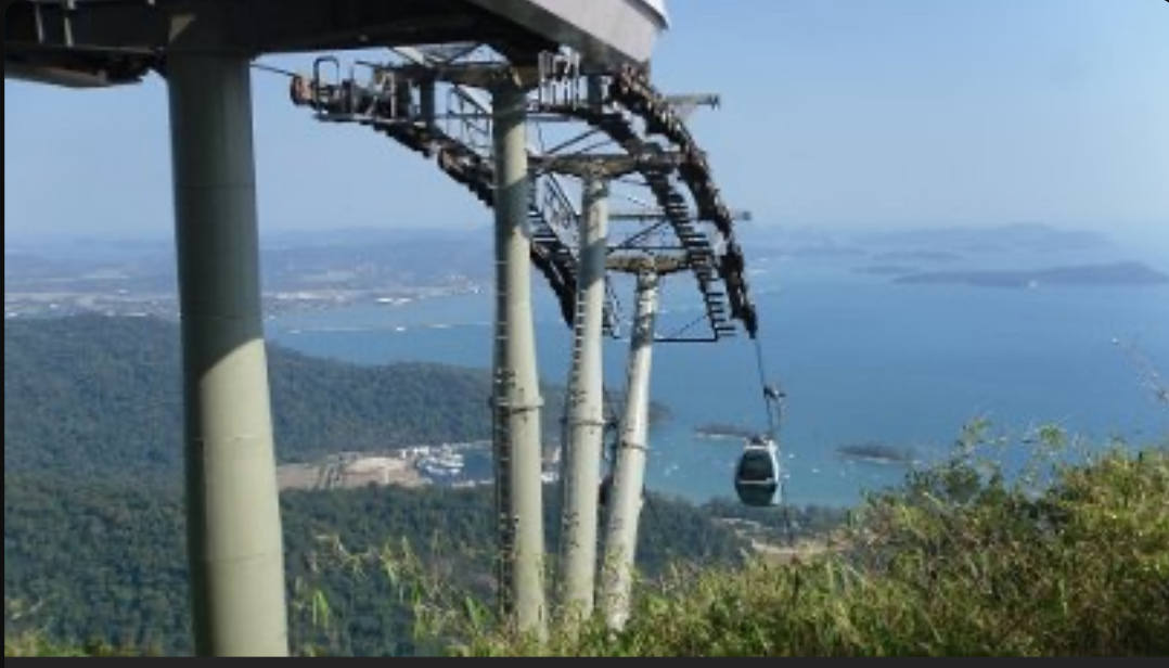
Cable car and pylons
