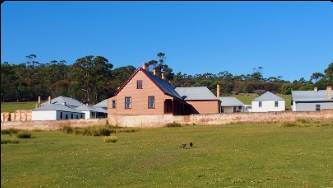
Darlington settlement buildings
