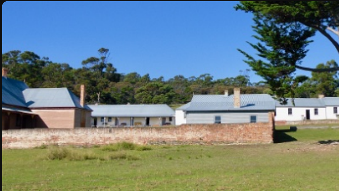
Darlington settlement buildings
