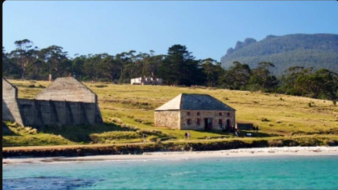
Remains of old cement works buildings, Darlington, with northern hills behind
