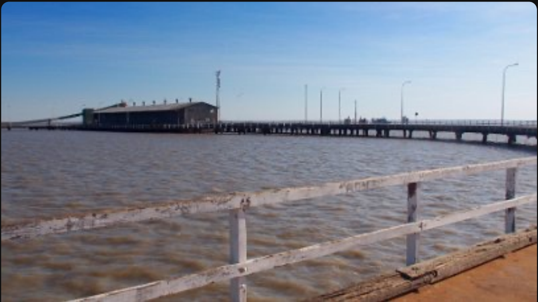
Circular jetty at Derby
