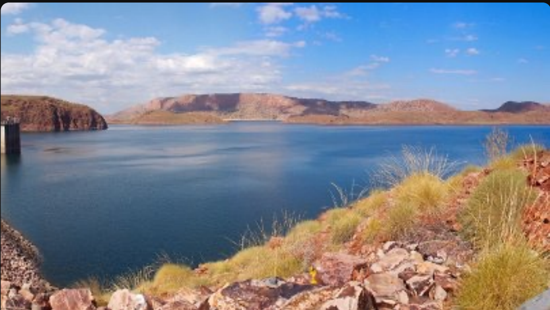
Lake Argyll and dam wall
