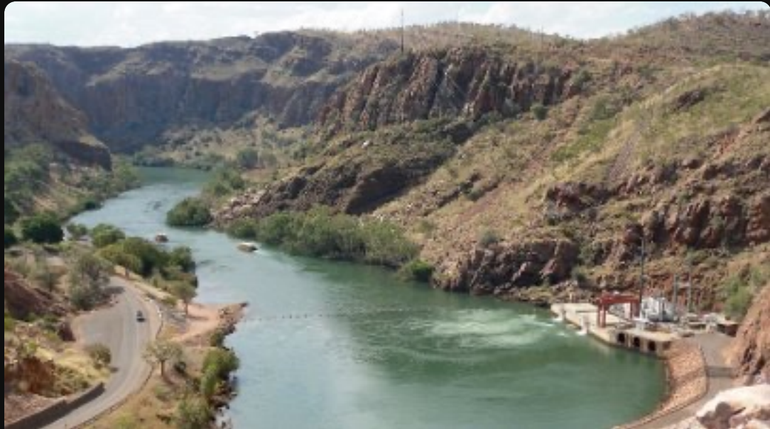
Downstream view from Lake Argyll dam wall
