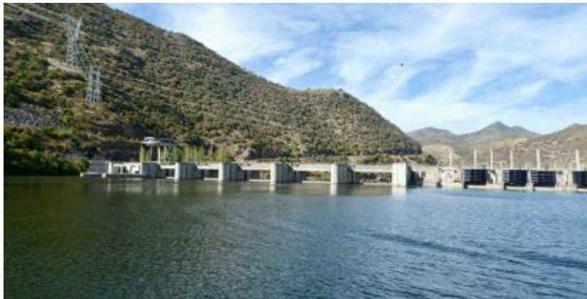
The Valeria Dam from its upstream side
