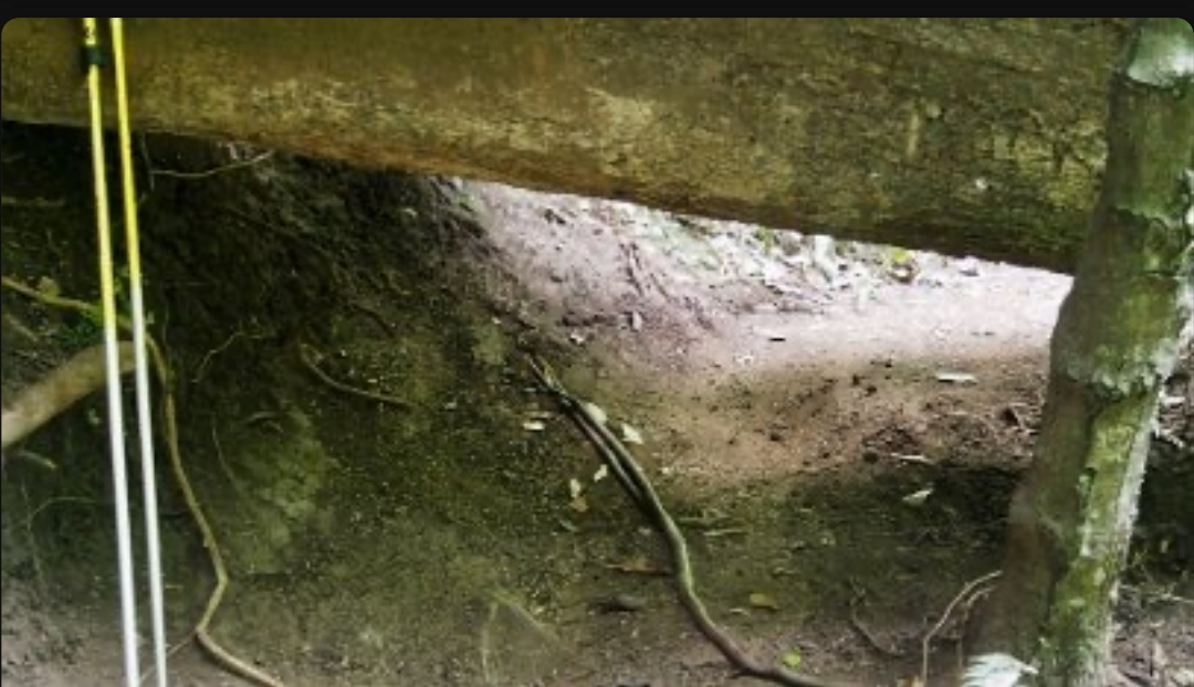
Low bridge under fallen tree
