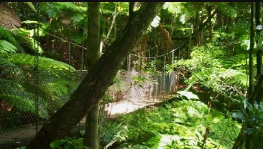
Suspension bridge across creek
