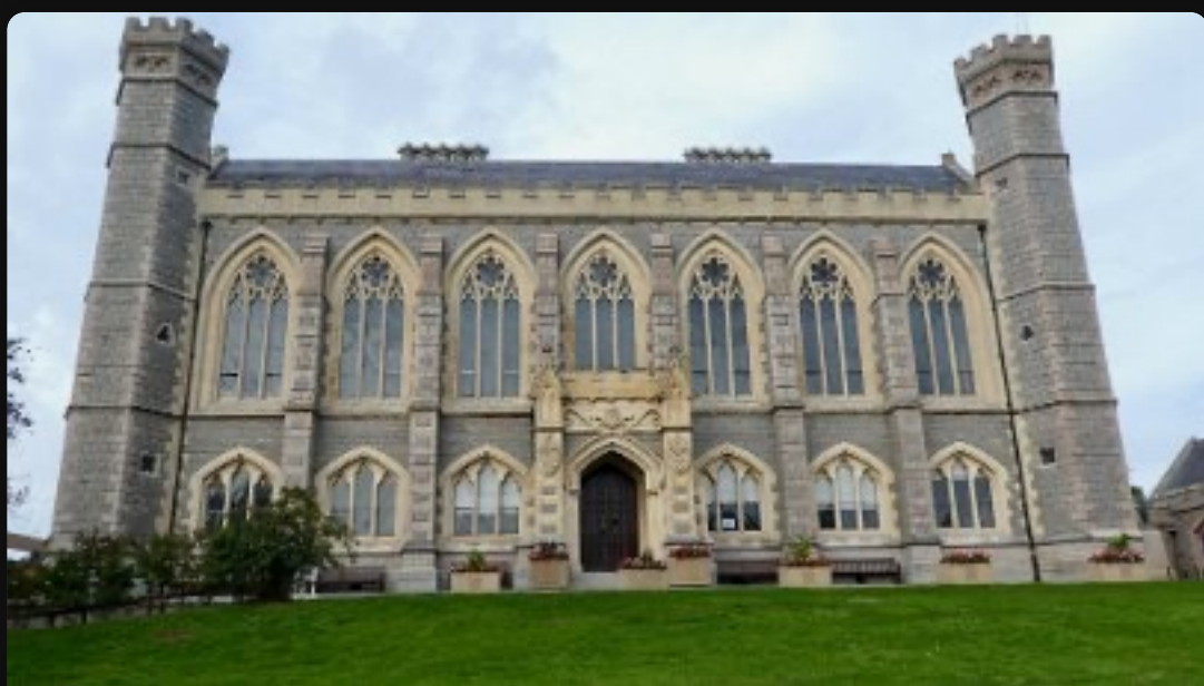
The main façade of Victoria College seen from below
