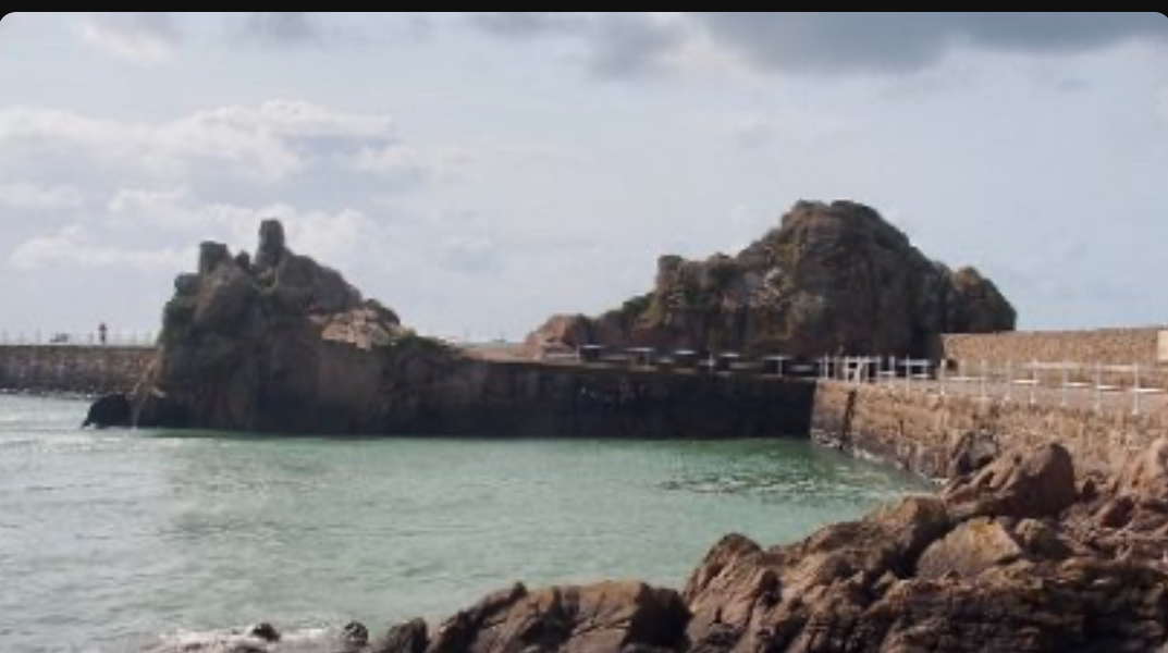
La Rocque Harbour and Breakwater
