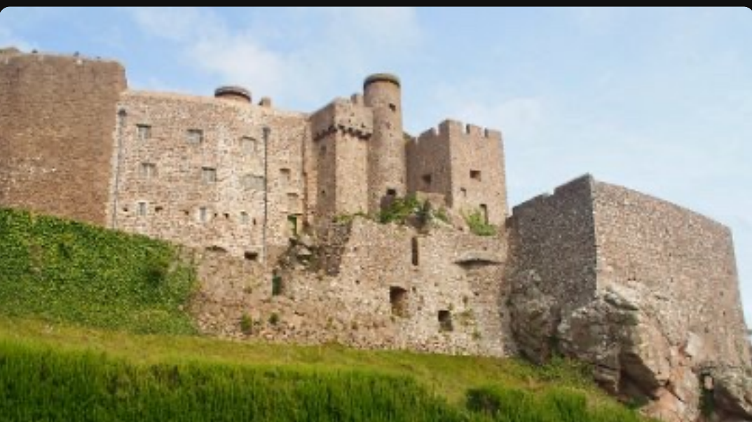
Mont Orgueil Castle upper levels
