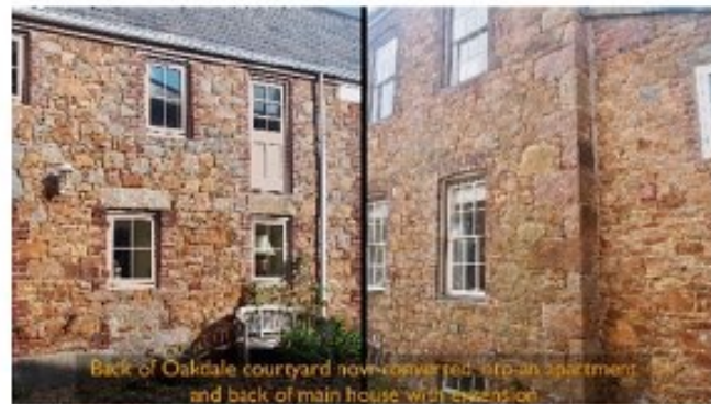
Back of Oakdale courtyard now covered with a wooden platform and back of main house with a new porch
