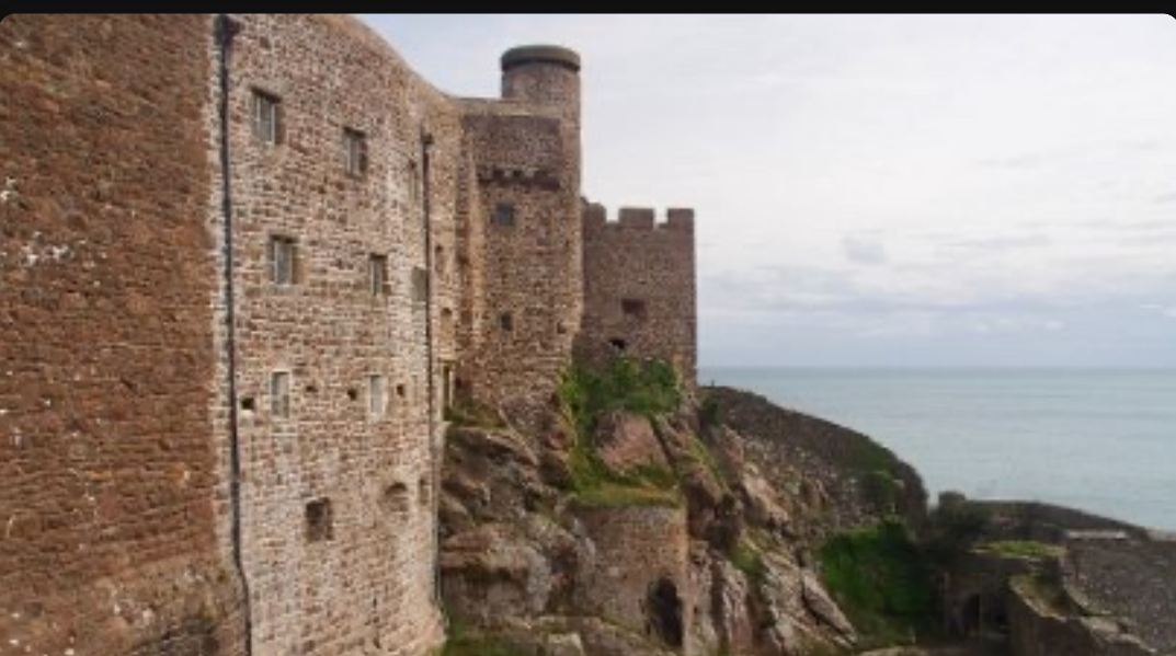
Mont Orgueil Castle showing part of mid level
