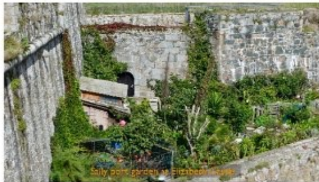
Tilly gate project at Elizabeth Castle
