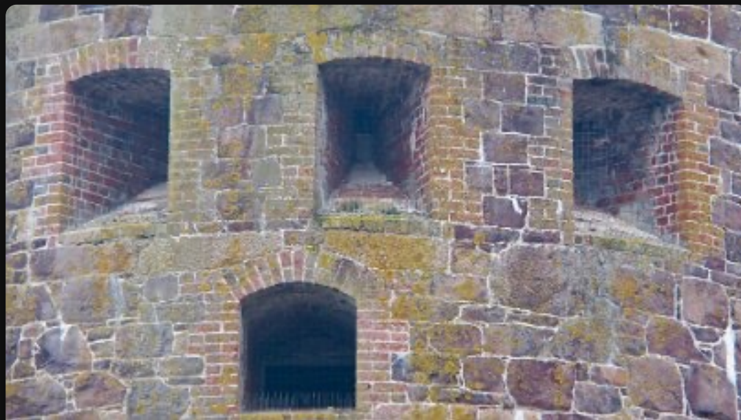
Window renovations at Archirondel Tower, St Catherine's Bay
