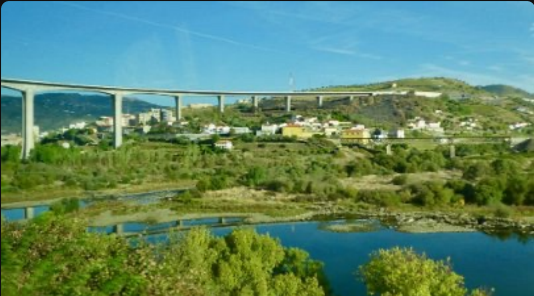
New A24 motorway bridge near Regua
