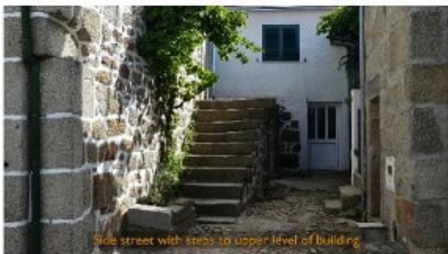
Side street with steps to upper level of building
