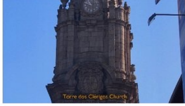
Torre dos Clerigos Church
