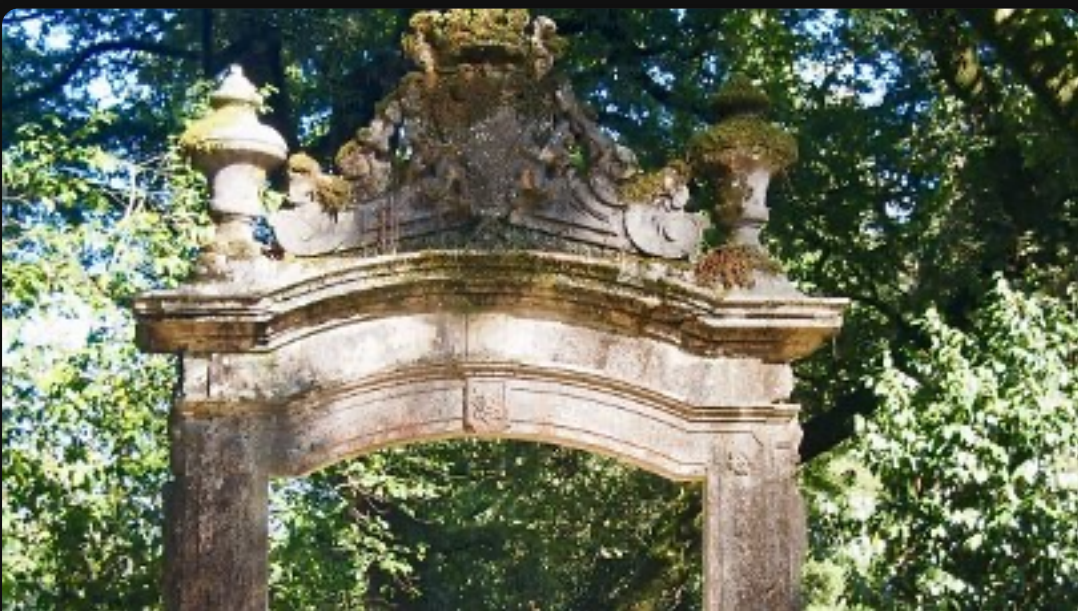
Old gate in gardens at Quinta da Aveleda Winery
