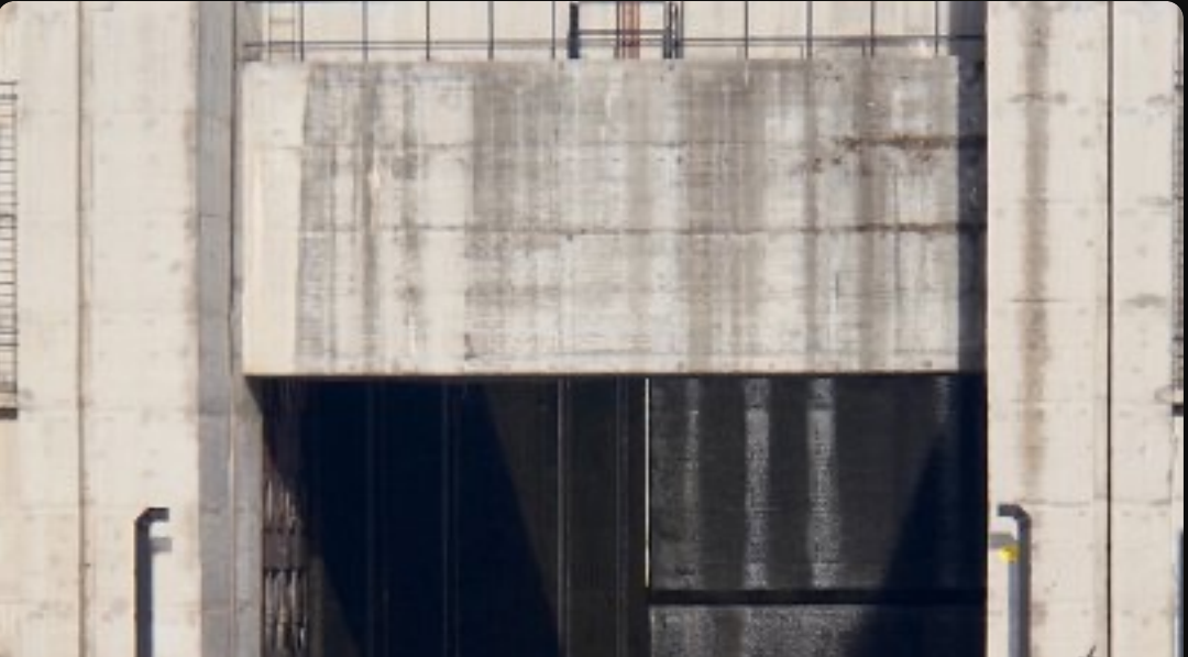
Entering the lock at Pocinho Dam
