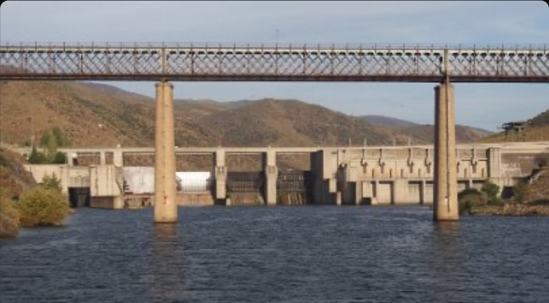
Approaching Pocinho Dam and railway bridge
