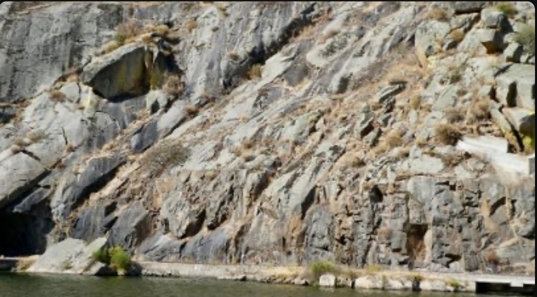
Steep rocky walls to Douro valley with a small space for a railway line
