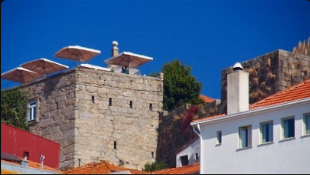
Part of old city wall near the Cais de Miragaia, Porto
