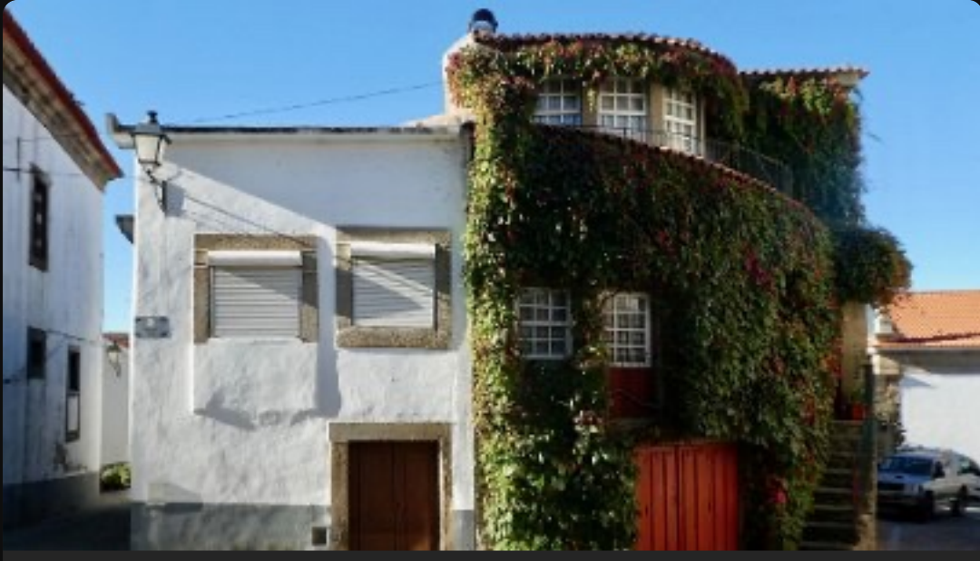
Renovated building on town square in Provesende
