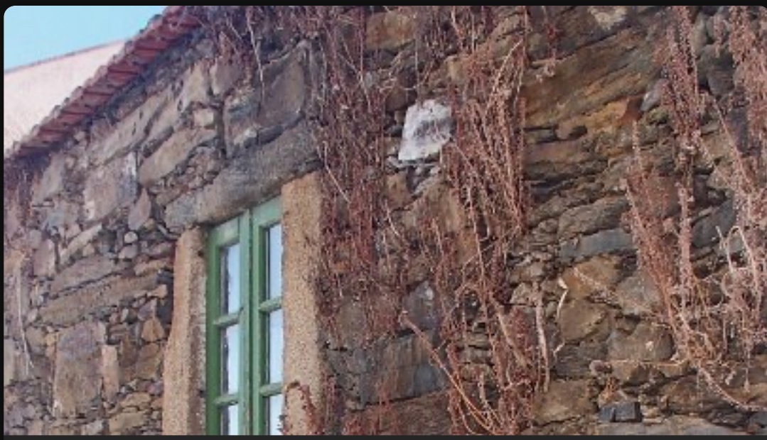
Building showing old wall in Provesende
