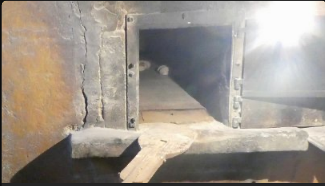
Town bakery oven in Provesende
