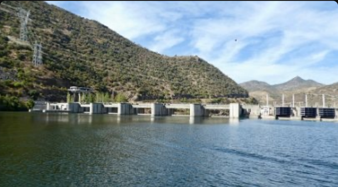
Upstream side of Valeira Dam
