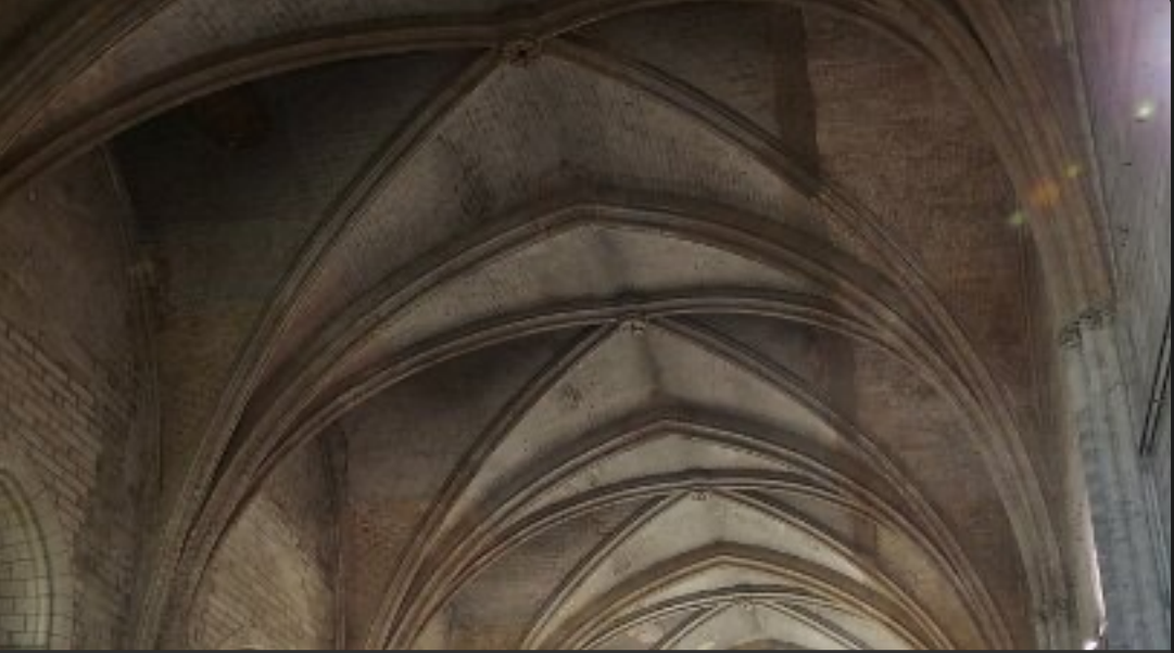
Roof of Grand Chapel with beautiful acoustics in Palace of the Popes, Avignon, Provence-Alpes-Côte d'Azur
