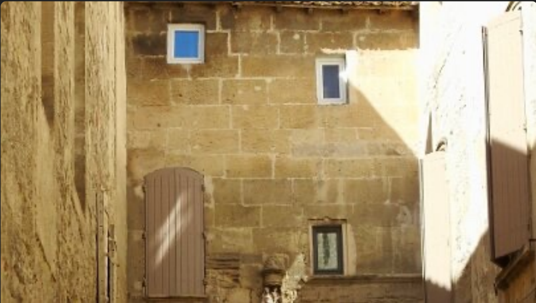
Passageway through to Boulevard Itam, Tarascon, Provence-Alpes-Côte d'Azur
