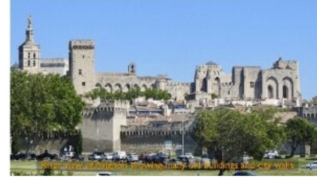
A view of the city of Avignon from the river.
