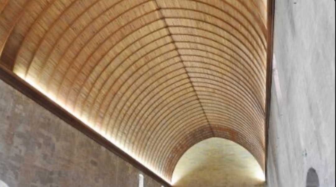
Barrel-vaulted roof of main dining room in Palace of the Popes, Avignon, Provence-Alpes-Côte d'Azur
