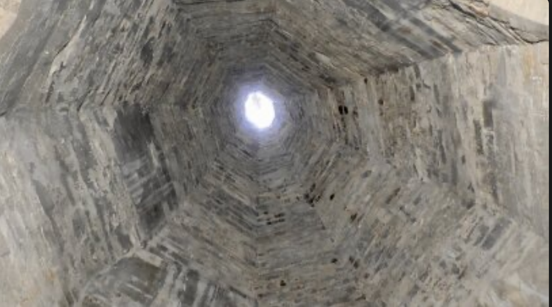
Conical roof to serving kitchen in Palace of the Popes, Avignon, Provence-Alpes-Côte d'Azur
