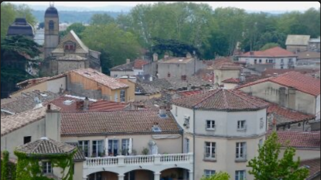
Roof top view of Tournon-sur-Rhône, Rhône-Alpes
