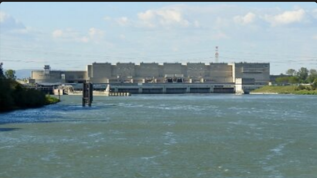
Leaving the hydro-electric station and lock at Les Tourrettes, Rhône-Alpes
