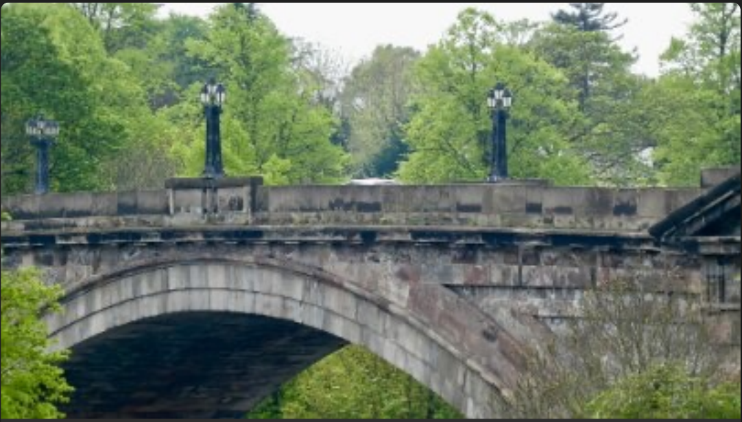
Grosvenor Bridge near Chester Castle, Chester
