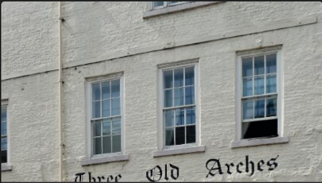
Three Old Arches, Bridge Street, Chester
