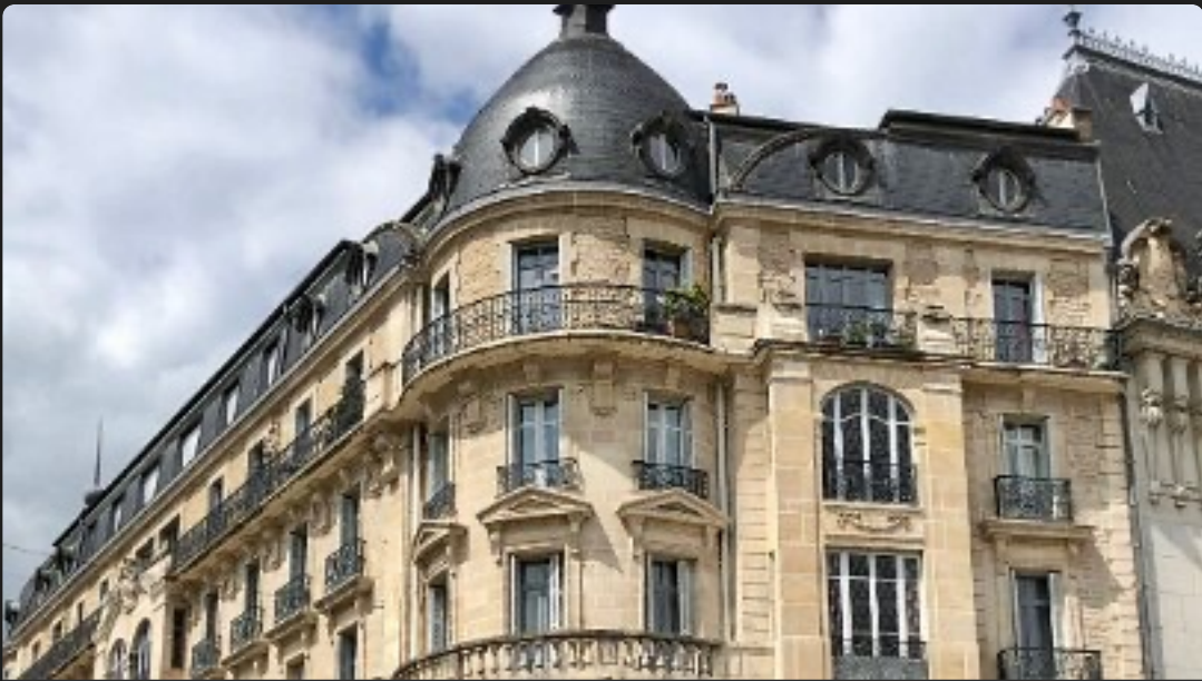
Corner of Rue de la Liberté and Place François Rude, Dijon, Burgundy
