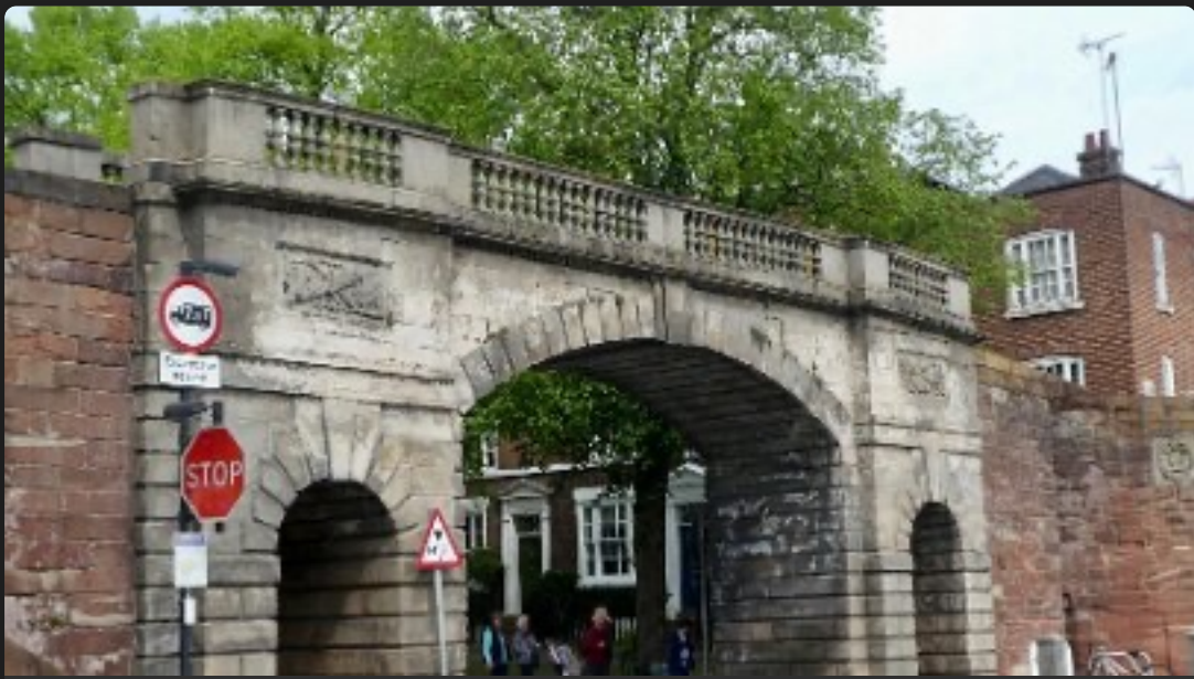
Wall crossing Bridge Street, Chester
