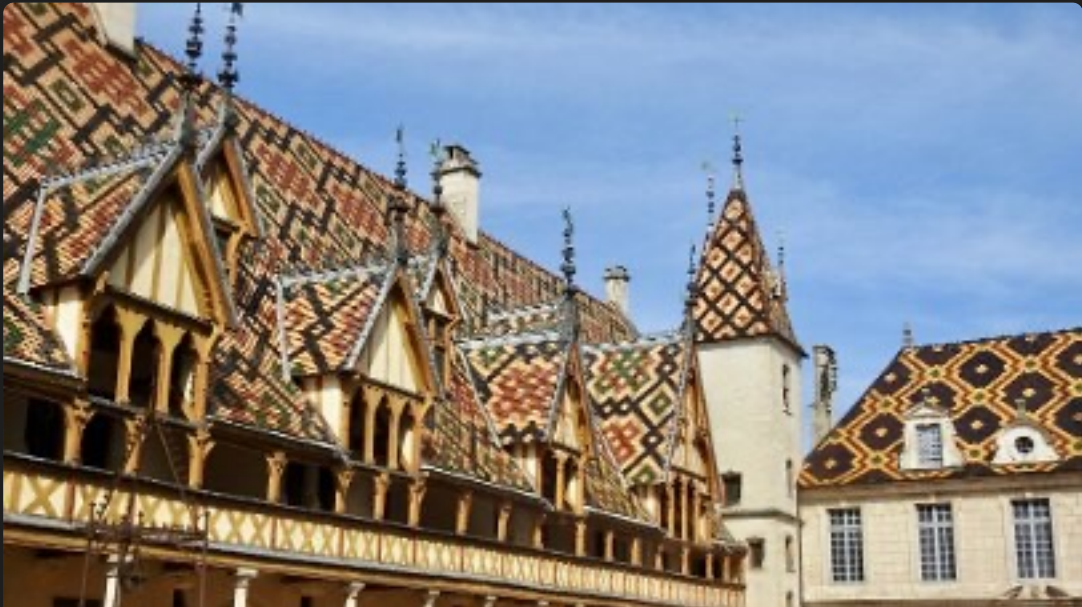
Courtyard view of roof of Hospices de Beaune, Beaune, Burgundy
