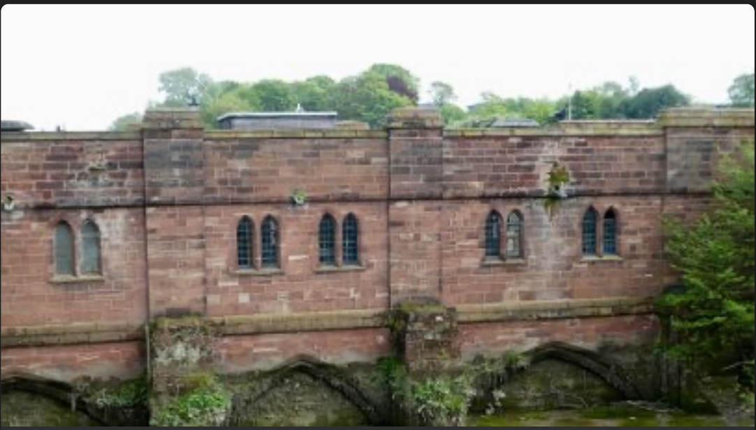
Part of Handbridge, the Old River Dee Bridge, Chester
