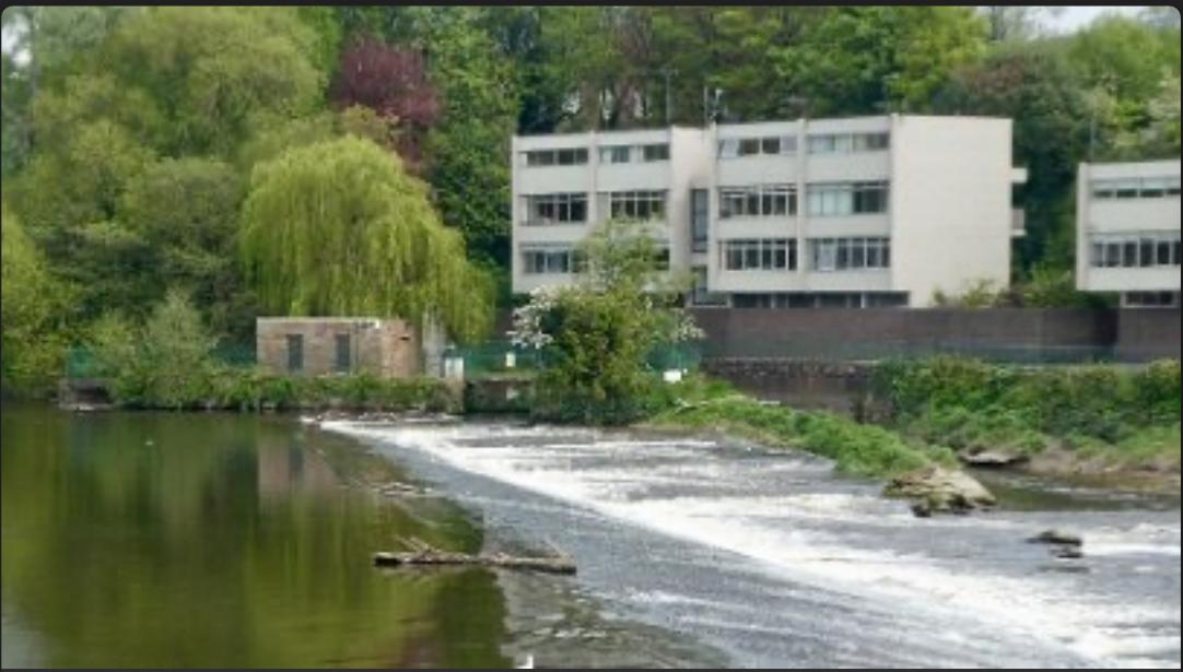
Weir on River Dee near Handbridge, Chester
