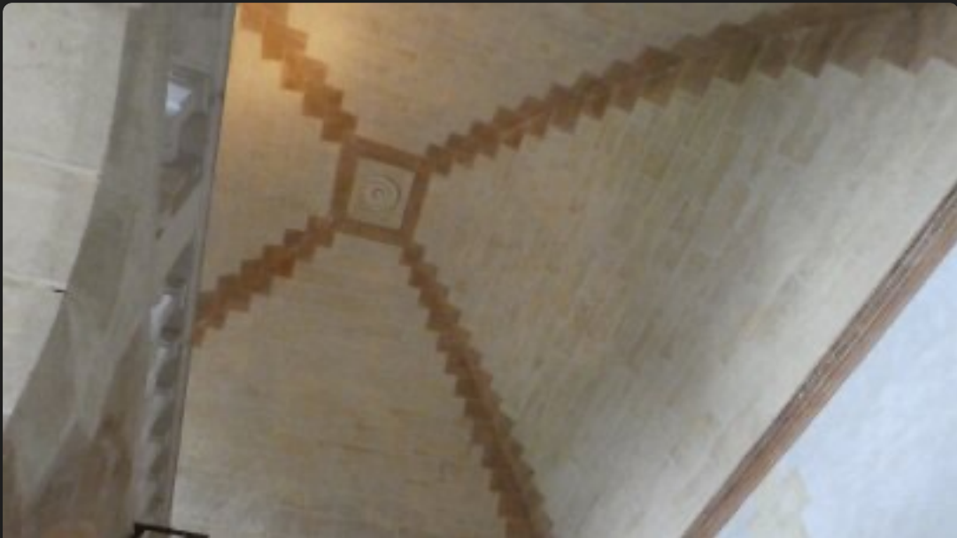
Staircase roof in Château de Cormatin, near Tournus, Burgundy
