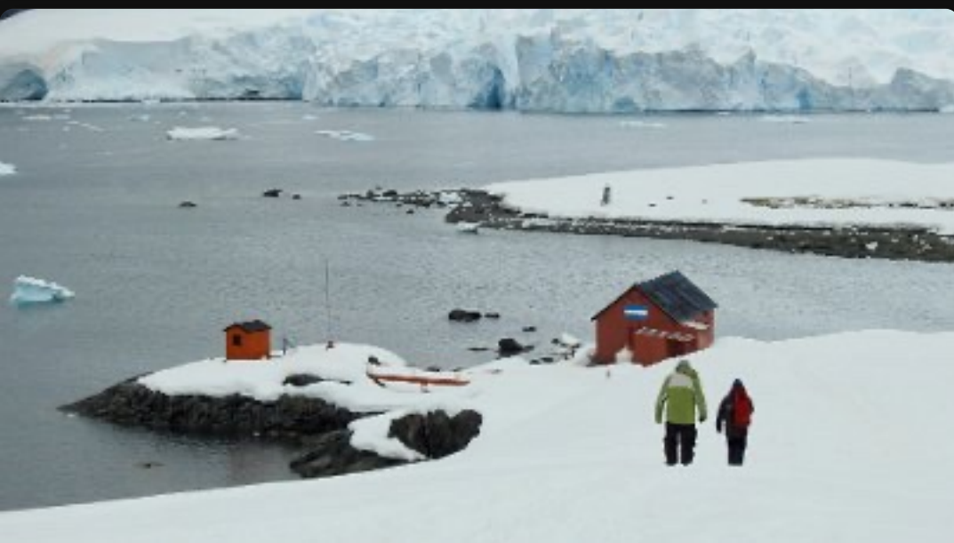
Looking down on Brown Station buildings
