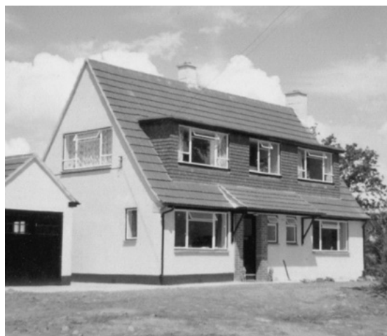
Building Little Coombe back (top left), front (top right) and completed (below), known as "Boom-boom's house", 1960
