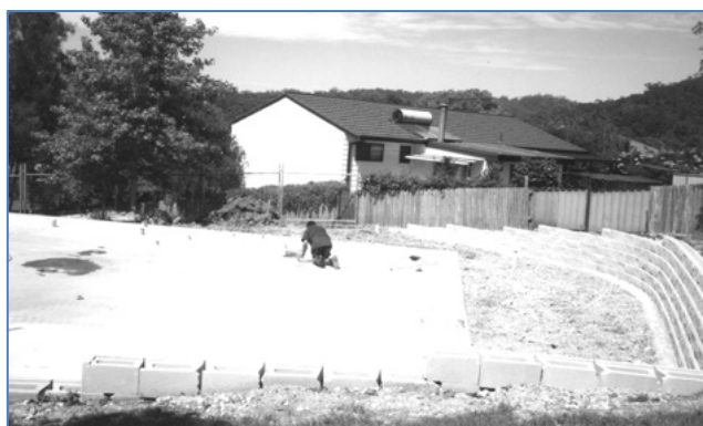
2005 Kendall: Foundations for RTC with retaining wall
