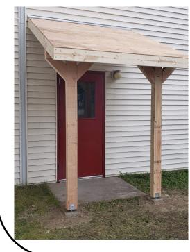
An awning roof has been built over the new exterior door to protect it from rain and falling ice. (This picture was taken before the metal roofing was added. The awning is now complete...but Melissa didn't get outside to take a picture before the snow arrived!)
