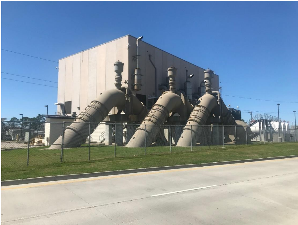
NEW SUPPLEMENTAL PUMP STATION DISCHARGE PIPES
