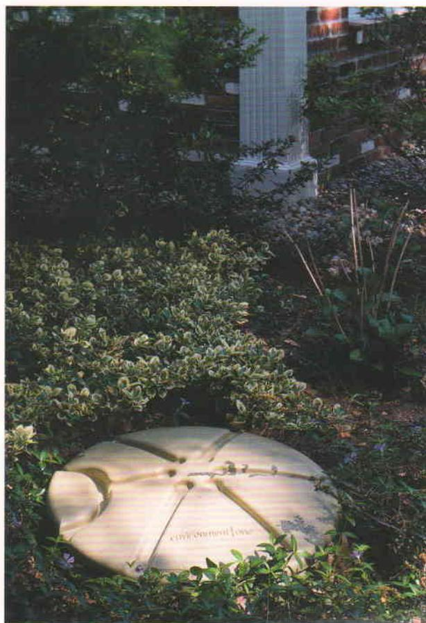
**If you go on vacation** for a length of time, flush the system before you go away. Run clean water into the unit until the pump activates. Turn off the water and allow the grinder pump to run until it shuts off automatically. If you have a duplex unit (two pumps), special attention must be taken to ensure that both pumps turn on when water is added to the tank.
