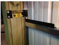
The Cincher controls the back side of the door and snugs the closed doors against the building.
