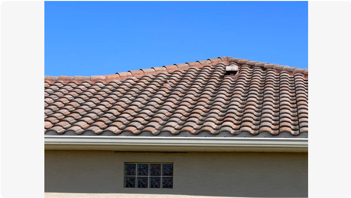
Photo of tiles on the roof
