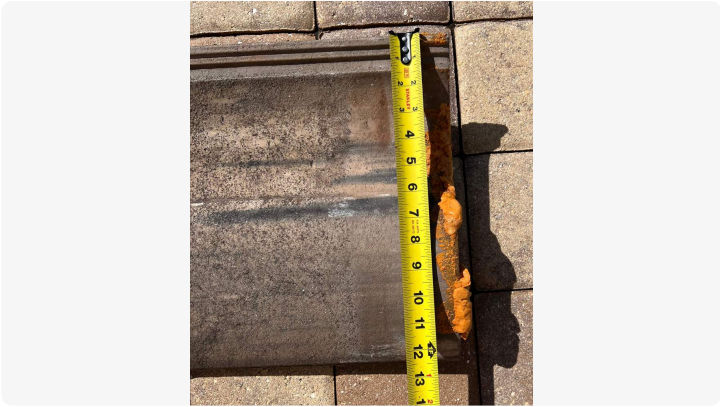
Measurement of top of tile
