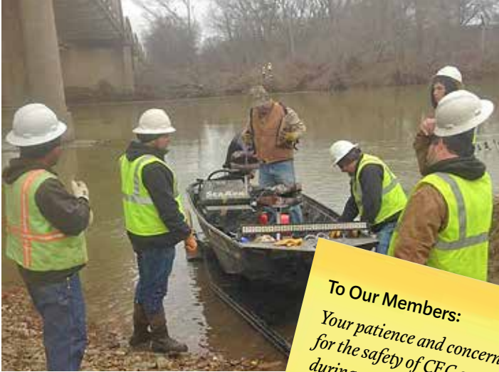
Choctaw Electric linemen prepare to ford the frigid waters of the Glover River following storms in December. Crew members raised 680 feet of submerged wire and reattached it to poles on either side of the stream. PHOTO/NORVIN GRAHAM
