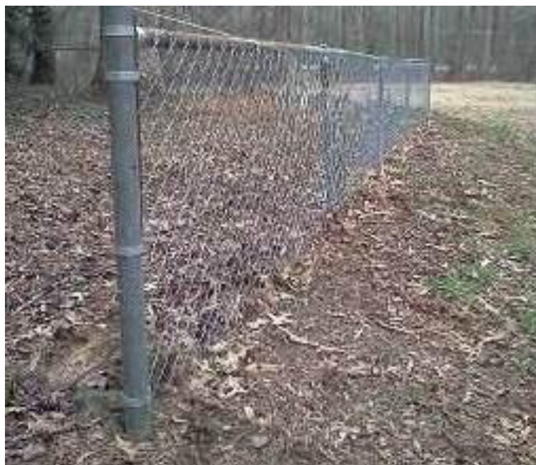
Fence repairs at Cowles-Spencer Cemetery
