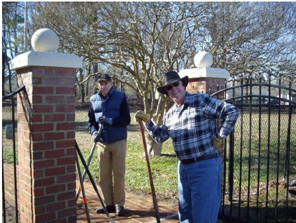
Ken Parsons and Ron Perry putting fill dirt along the edges of the sidewalk.
