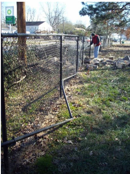
Dennis Dasher repairs the fence.
