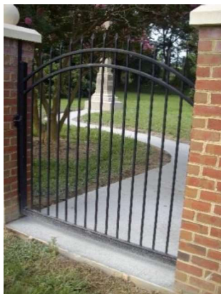
In July, Chuck Mihalcoe and ABBA Concrete poured the base for the walkway from the gate to the Soldier & Sailor's Monument.
