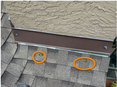
Fasteners are sealed, but this is incorrect
