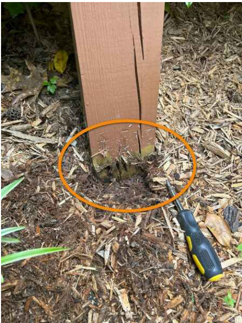
No Footer, Some Rot, Back Right Deck
