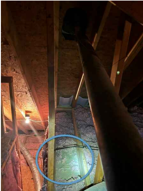
Missing insulation
