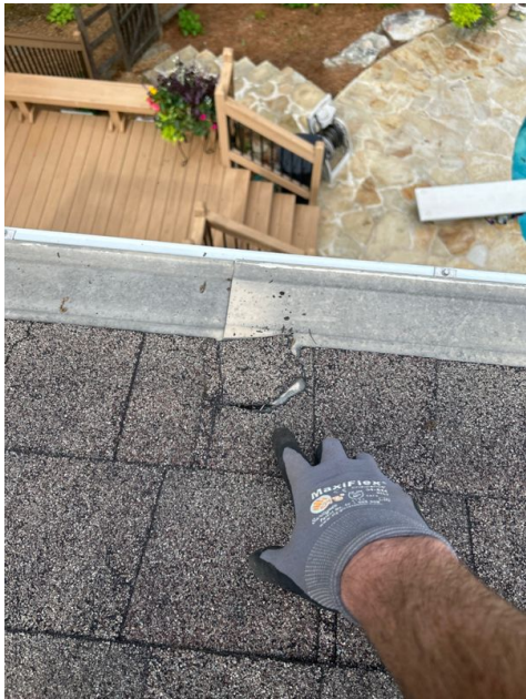
Fasteners are sealed, but this is incorrect
