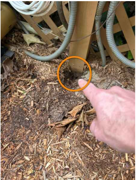
No Visible Footer, Some Rot, Back Left Deck.
