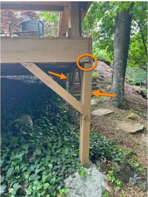
Important: Correct Support Post. Leaning. Back Left Deck
