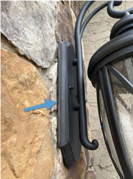
Recommend sealing all exterior lights
