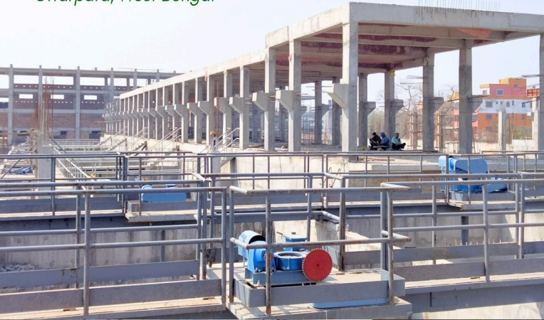
Final cover slab RGSF pipe gallery 250MLD WTP project Uttarpara, West Bengal
