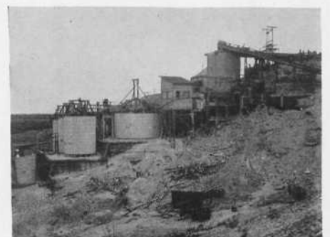
Holmes and Nicholson plant near Winterhaven, Imperial county, California.
