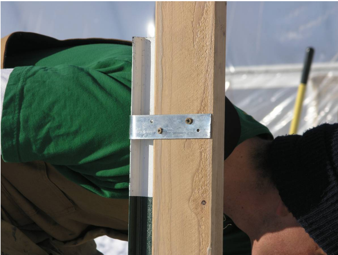
Attatch end wall to t-posts with plumbers strapping Return to Text
