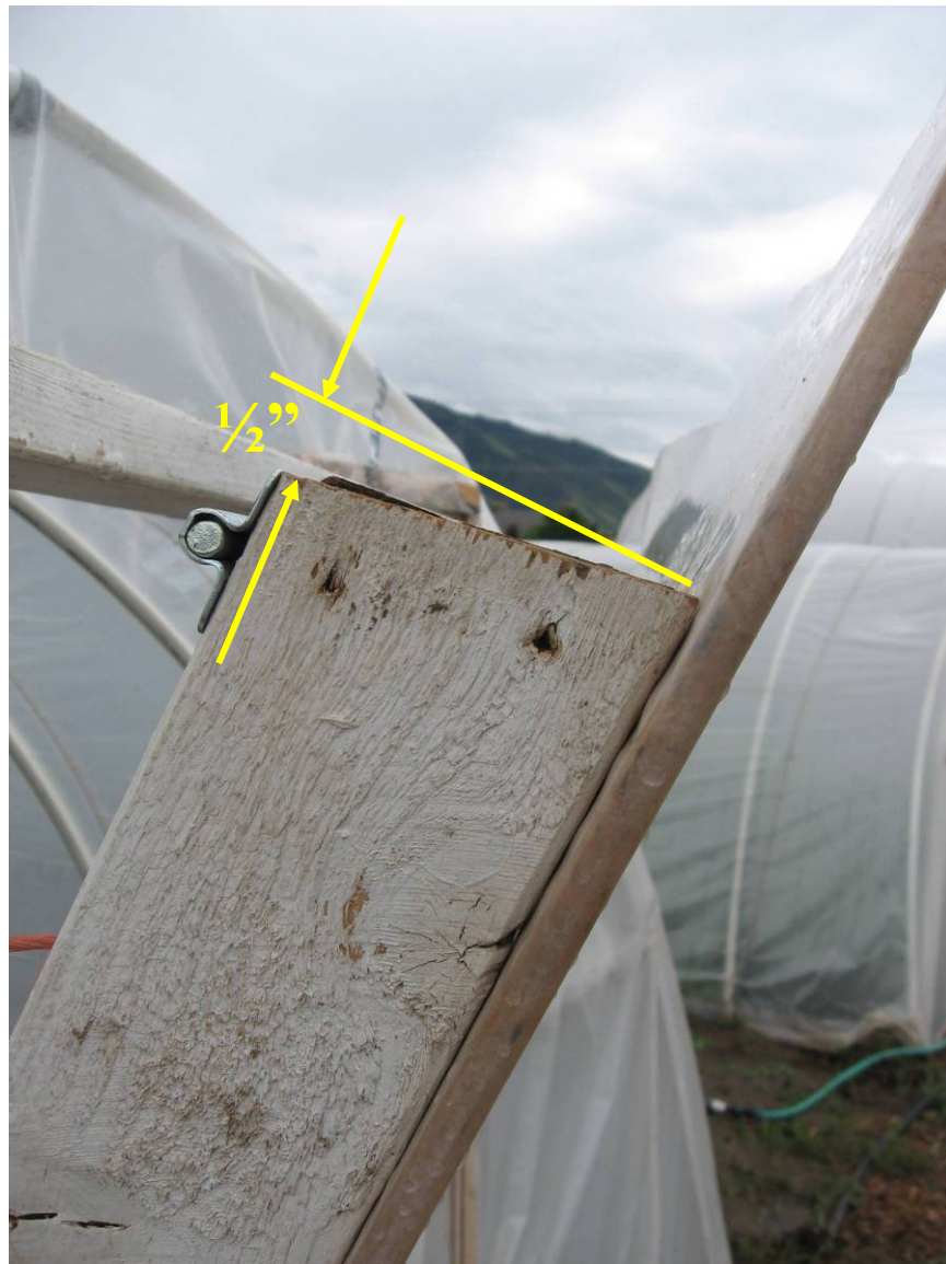
Side view of top venting door with 1/2" bevel on top vent
