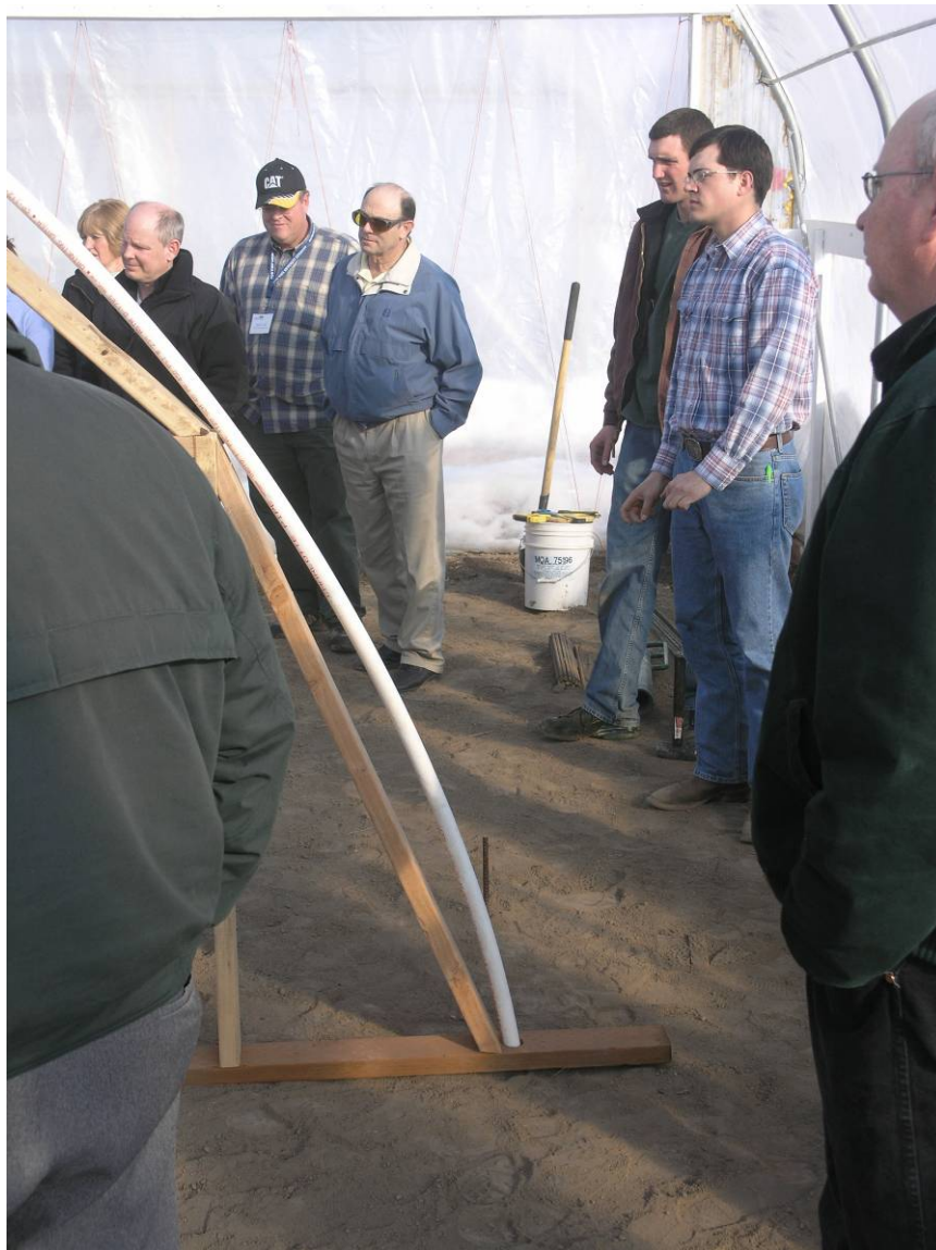
PVC pipe slides into 1 1/4" drilled holes
