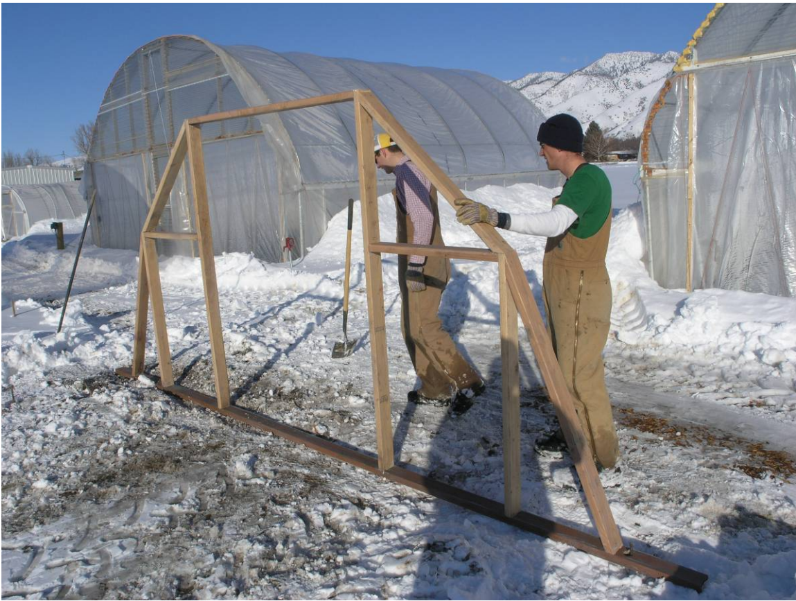
Pre-Constructed End Wall Return to Text
