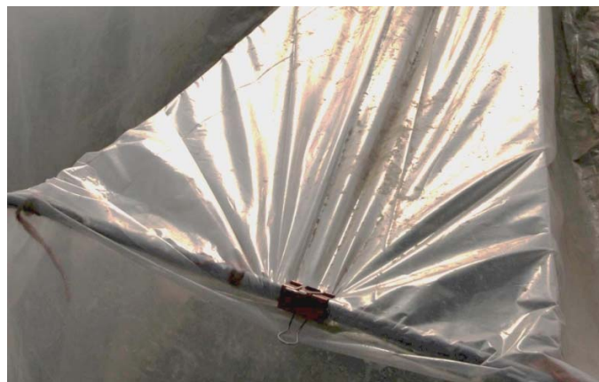
Image 7. Binder clip securing plastic to conduit frame.
