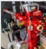
Elkhart valves with ball control handles on a painted stainless steel manifold
