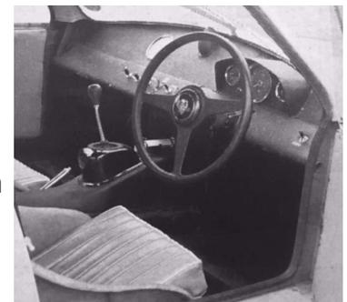
riding switch for the fuel pump. The speedometer is ahead of the passenger seat and a fire extinguisher is mounted in a clip on the gearbox tunnel.
