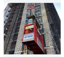
Among other applications, construction hoists are typically used on construction sites with high requirements for the transport of people and materials, in the construction of high-rise buildings and bridge pylons. STROS hoists are designed and manufactured for long life and reliability.
