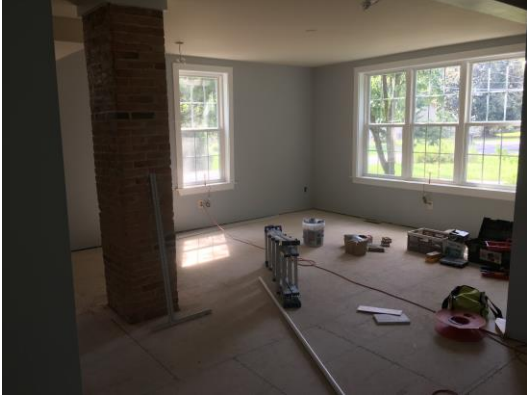
Former living room with exposed chimney
