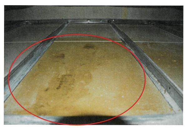
49. A large section of the ceiling sheetrock was removed and seized, which included the stain, metal framing, and the hole for the ceiling vent. The ceiling vent itself was also seized. The photo below shows the area of sheetrock and metal framing that was seized; the area of staining is again circled.
