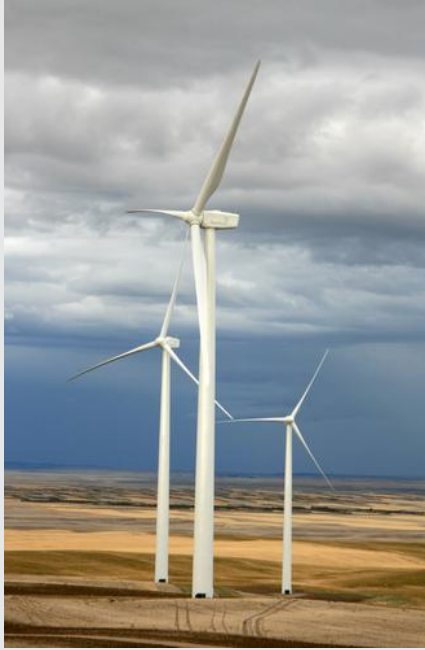
Wind turbines in Montana. Photo: Obel Kraus/NREL
