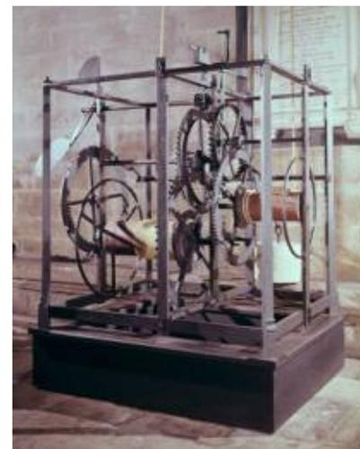
At the end of the 17<sup>th</sup> century, along with many other clocks of that era, the clock's verge and foliot escapement was replaced with a more accurate pendulum and recoil escapement. The 1956 restoration project returned it to its original design. Today, though the striking mechanism is silenced, the clock runs as it did over 600 years ago 🕒
