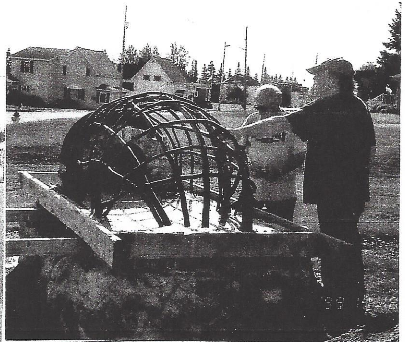
Alder Branches Shaped to Form the Inner Shell of the Oven
