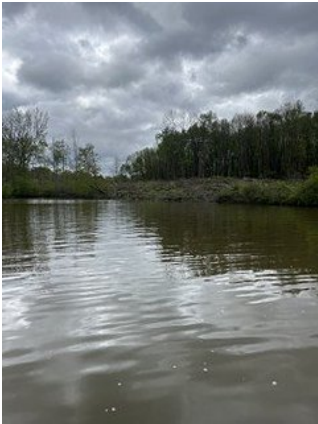
Tree removal near southern Hawthorn channel
