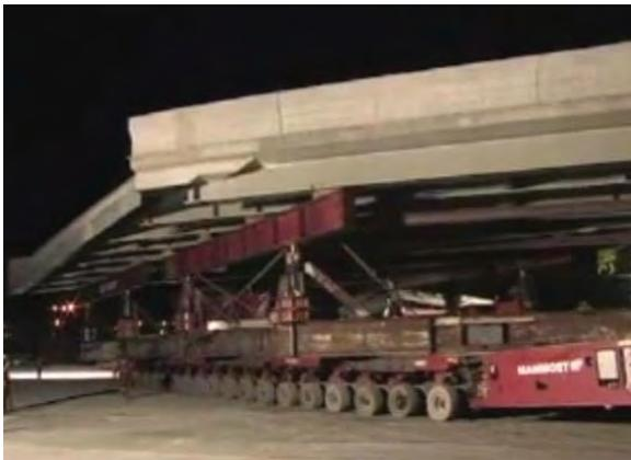
Figure 16: SPMT Moving a New Prefabricated Superstructure
