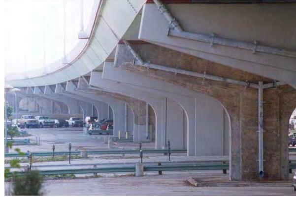
*Figure 10: Replacement of Drains and Coating Application*
