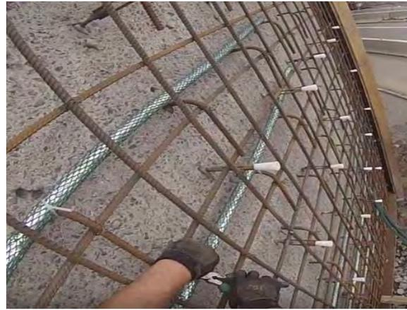
Figure 15: Distributed Galvanic Anodes and Additional Reinforcing Steel
