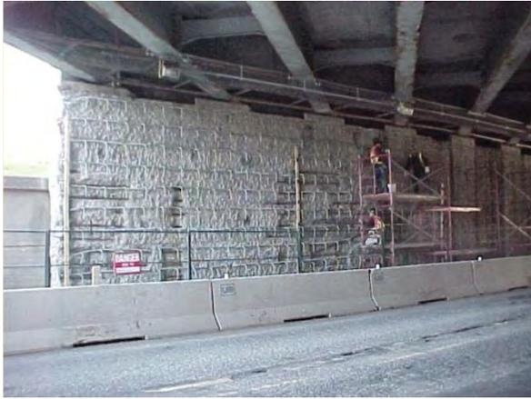
Figure 14: Re-facing of Existing Abutments
