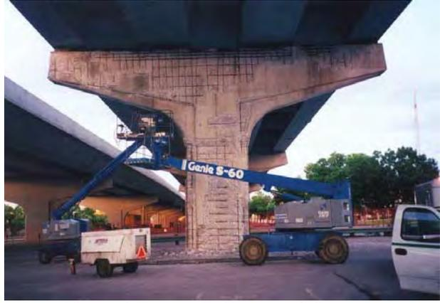
Figure 4: Removal of Damaged Concrete
