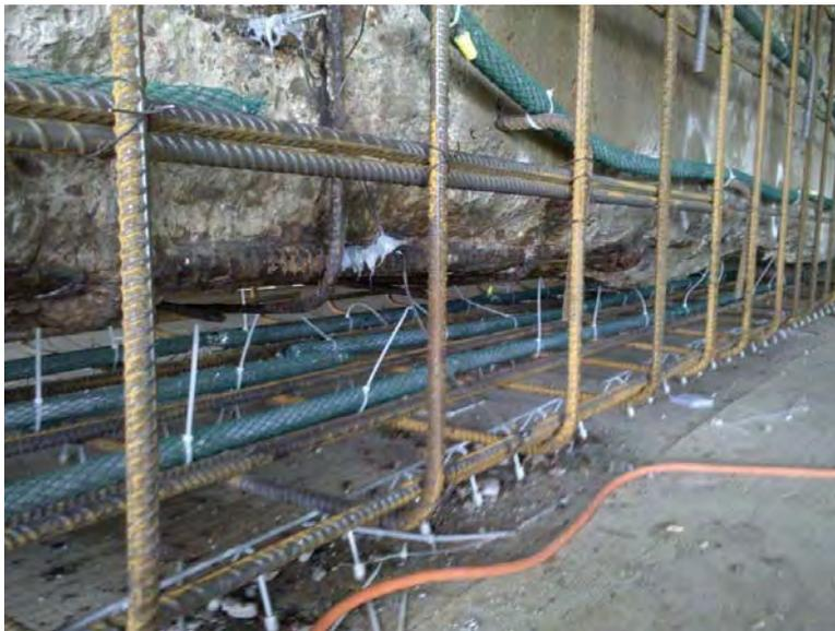
*Figure 2: Pier Cap Repair Using Reinforced Concrete Encasement with Distributed Galvanic Anodes, George Wade Memorial Bridge Rehabilitation, 2011*
