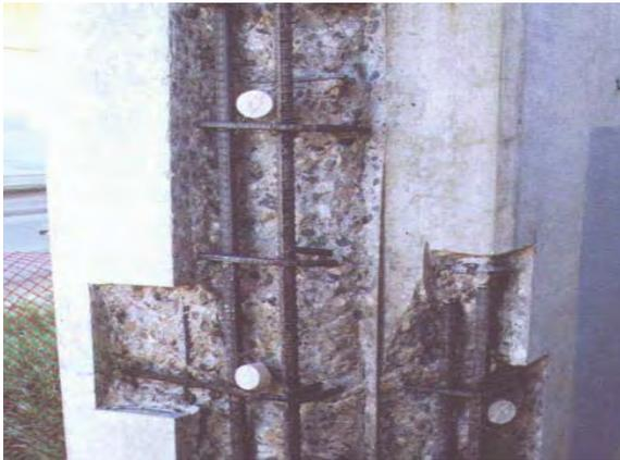
Figure 5 Patch Repair with Type 1A Anodes
