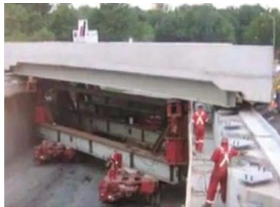
Figure 17: New Superstructure In-place
