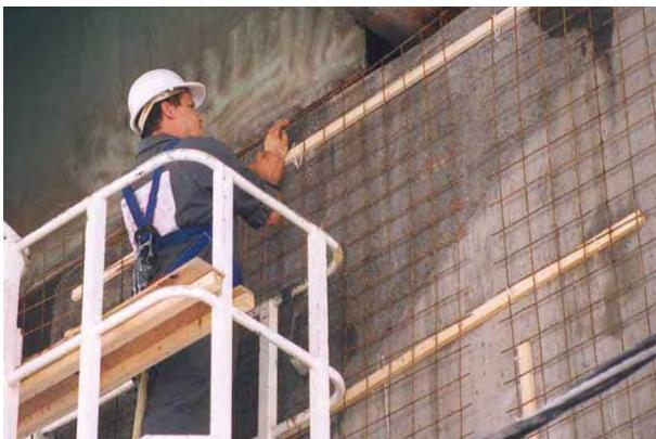
Figure 7: Temporary Anode Placement
