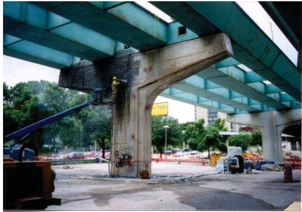
Figure 6: Concrete Repairs
