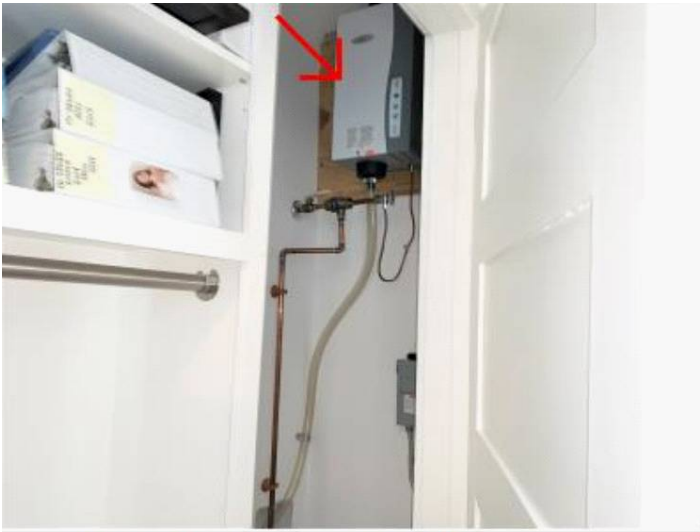
humidifier equipment/improperly installed
