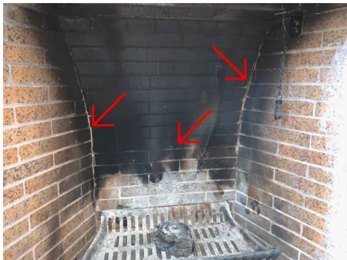
cracking masonry
