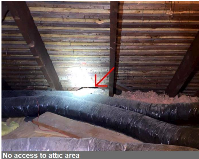
No access to attic area
