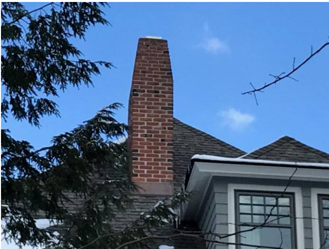
chimney is located at the left, rear
