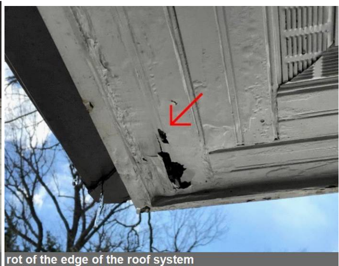
rot of the edge of the roof system
