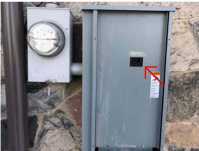
200 ampere primary panel board
