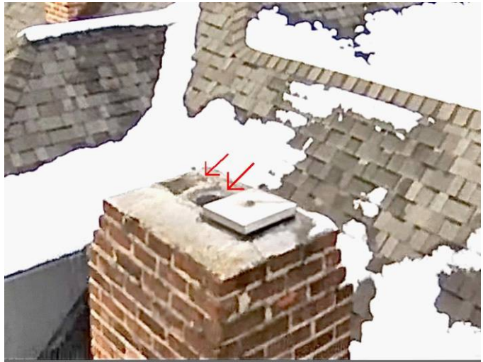
chimney caps are NOT installed
