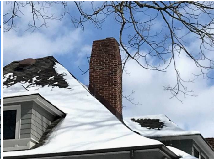
chimney is located at the left, rear
