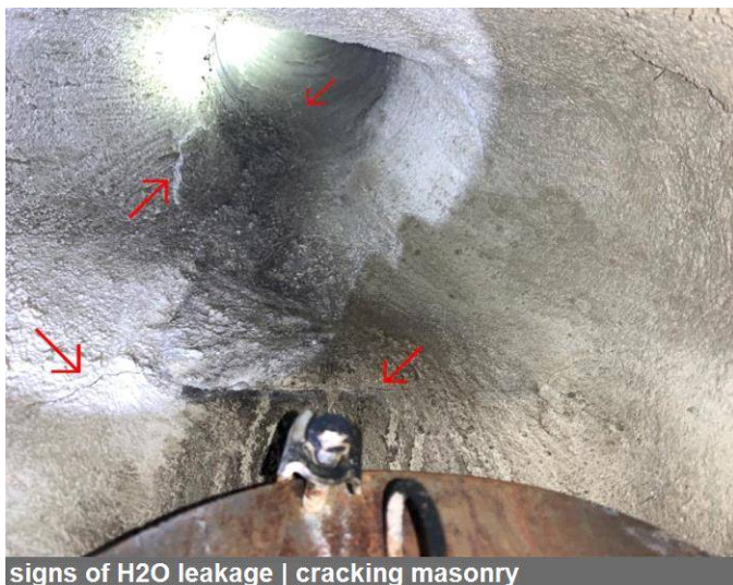
signs of H2O leakage | cracking masonry
