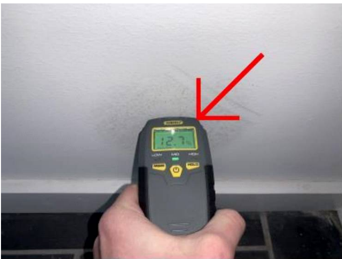
staining consistent with leakage
