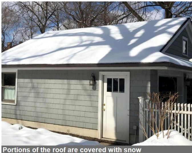
Portions of the roof are covered with snow
