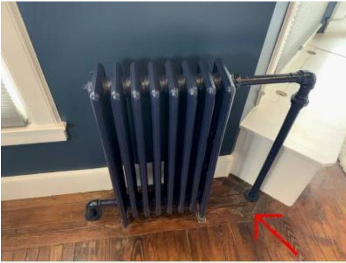
Damaged flooring (signs of leaks)
