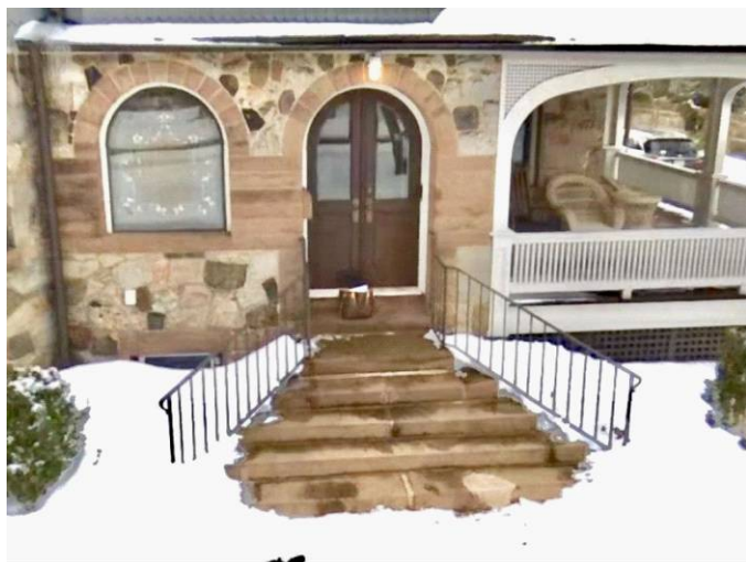
front porch | snow prohibits full view
