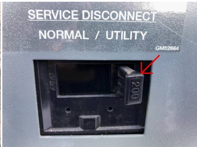
200 ampere primary panel board
